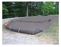
Compost mulch used as a ground cover and as a fill in a check dam.
