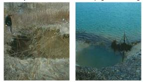
A large sinkhole on the downstream slope and the corresponding sinkhole on the upstream slope at the waterline next to the spillway inlet. SEEPAGE
