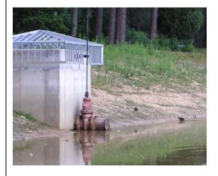
To test a valve or gate without risking that the lake will be drained, one must somehow physically block the drain inlet upstream from the valve. Some drain structures have been designed with this capability and have dual valves or gates, or slots for stoplogs (sometimes call bulkheads) located upstream of the
