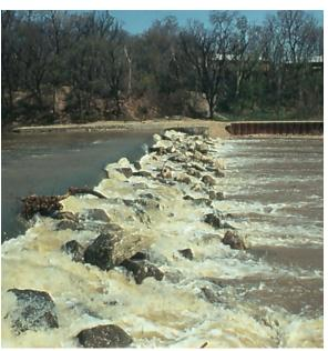
Large rock used to break up roller.
