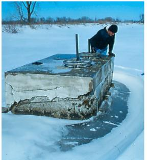
adjacent surfaces must be flush or the downstream one slightly lower to prevent erosion of the concrete, and to prevent water from being directed into the joint during high velocity flow. All joints should be kept free of vegetation. All weep holes should be checked for blockage, and concrete stain outlines on concrete surfaces studied for an indication of flow characteristics.
