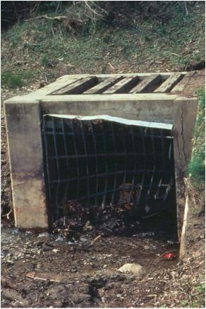
The trashrack should be properly attached to the riser inlet, and strong enough to withstand the hammering forces of debris being carried by high velocity flow, a heavy load of debris, and ice forces. If the riser is readily accessible, vandals will throw riprap stone into it. To prevent such vandalism, the size of the trashrack openings should not be decreased, but rock that is larger than the openings or too large to handle should be used.
