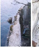
Structural problems are indicated by cracking, exposed reinforcing bars, large areas of broken-out concrete, misalignment at joints, undermining and settlement. Rust stains may indicate internal rusting and deterioration of reinforcement steel. Spillway floor slabs and upstream slope protection slabs should be checked for undermining (erosion of base material).
