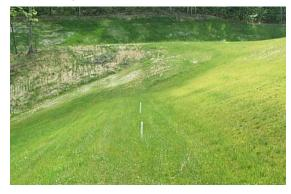
Settlement monuments - Settlement monuments are usually installed along the crest of the dam to check its vertical and horizontal alignments (with known reference points and elevations) Measurements of these monuments must be precise and are obtained using surveying instruments.
