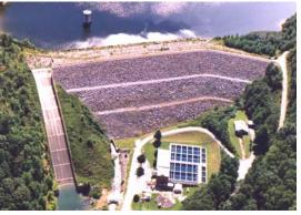
An embankment with associated works (principal spillway, emergency spillway and lake drain control tower).
