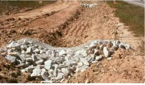
rock check dams across the gully until permanent repairs can be made can slow erosion in large gullies.
