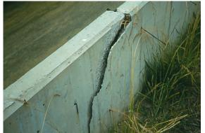
Before attempting repair of a concrete surface, all unsound concrete should be removed by sawing or chipping, and the patch area thoroughly cleaned. A sawed edge is superior in every way to a chipped edge, and sawing is generally less costly than mechanical chipping.
