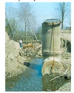
erode soil from the embankment or its foundation, resulting in rapid failure of the dam. Erosion of the soil begins at the downstream side of the embankment, either in the dam proper or the foundation, progressively works toward the reservoir, and eventually develops a "pipe" or direct conduit to the reservoir. This phenom-
