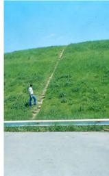
Not only should the eroded areas be repaired, but also the cause of the erosion should be addressed to prevent a continuing maintenance problem. Erosion might be aggravated by improper drainage, settlement, pedes-trian traffic, animal burrows, or other forces. The cause of the erosion will have a direct bearing on the type of repair needed.
