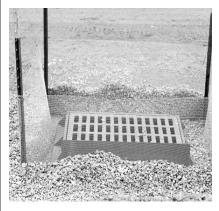
The North Carolina Department of Transportation's Roadside Environmental Unit discovered that the conventional inlet protector BMP can be improved by replacing the silt fence perimeter guard with a wire cage. The wire cage is sturdy and rigid and doesn't get weighed down by runoff and sediment like silt fence can.
