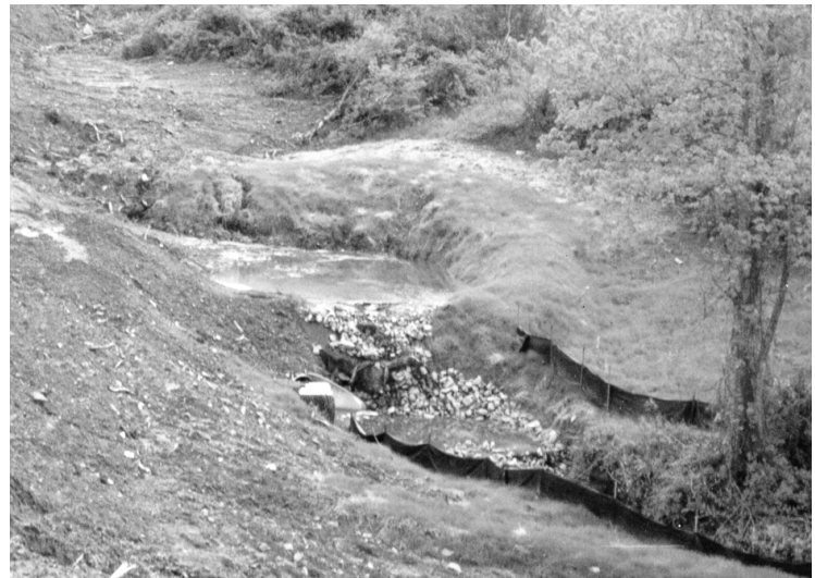
A sediment trap is a small temporary ponding basin formed by an embankment or excavation. Water is released from a sediment trap through a washed stone outlet.
