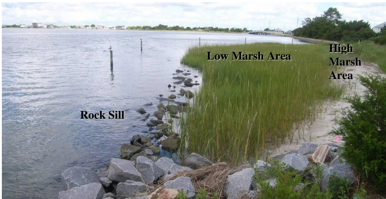
Figure 3: DUML restoration site with features labeled. Style of old bulkhead can be seen in distance.
