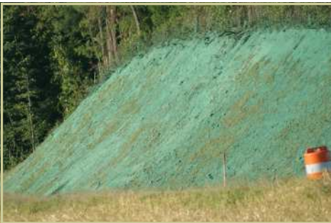
HECPs: Pictured above is a slope which has been stabilized with hydraulic applied product.
