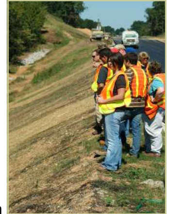
US 52 in Stanly Co: Project review with NCDOT, Land
