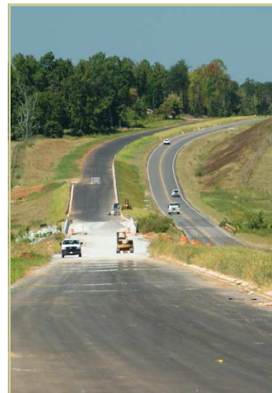
Linear Construction: US 70 project in Rowan county.
