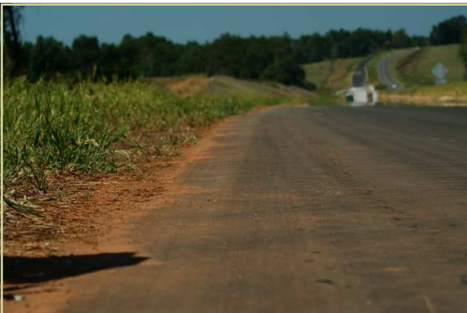
Stabilized Shoulder: US 70 in Rowan County
