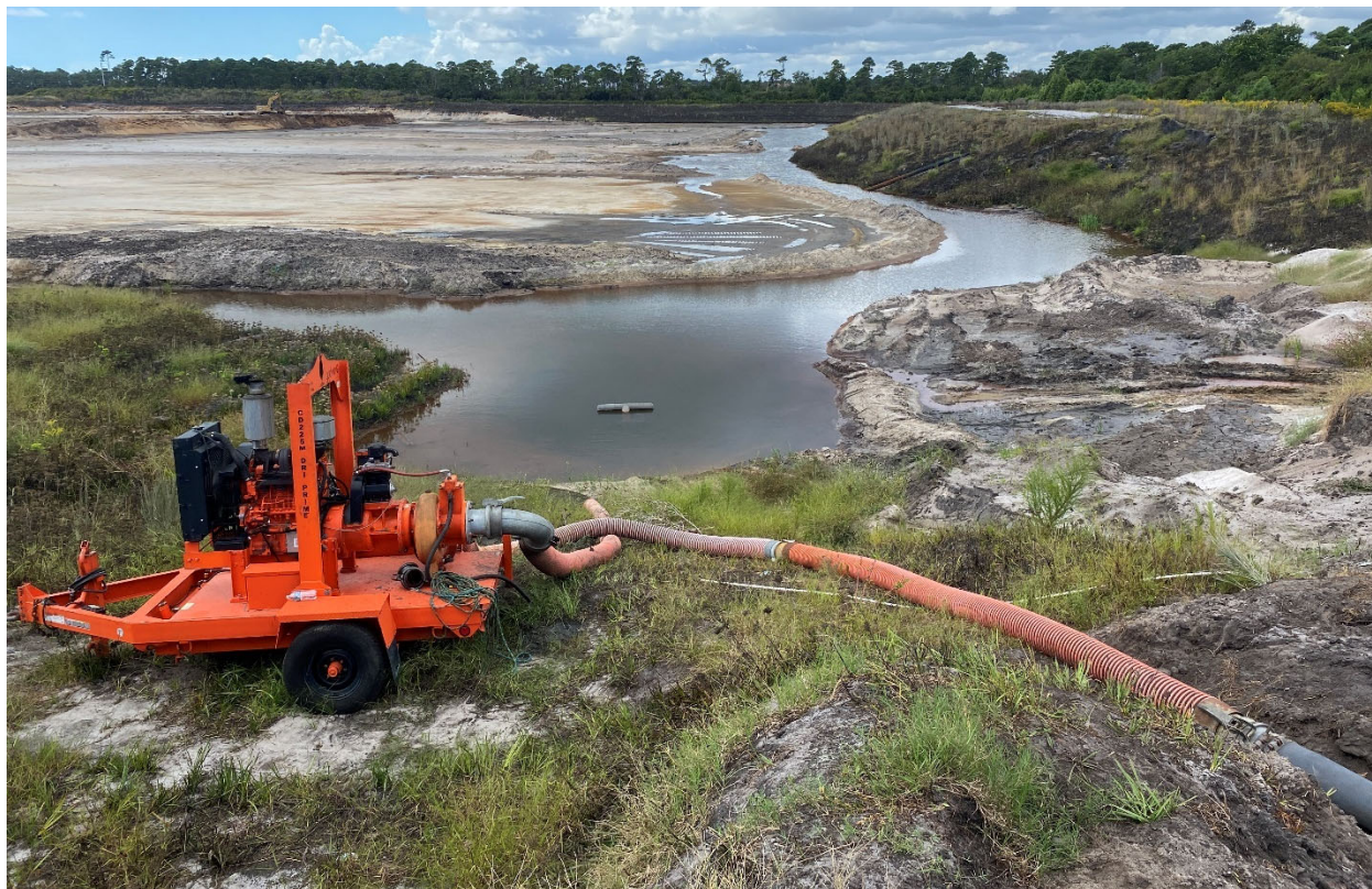
Borrow site pit actively dewatering.
