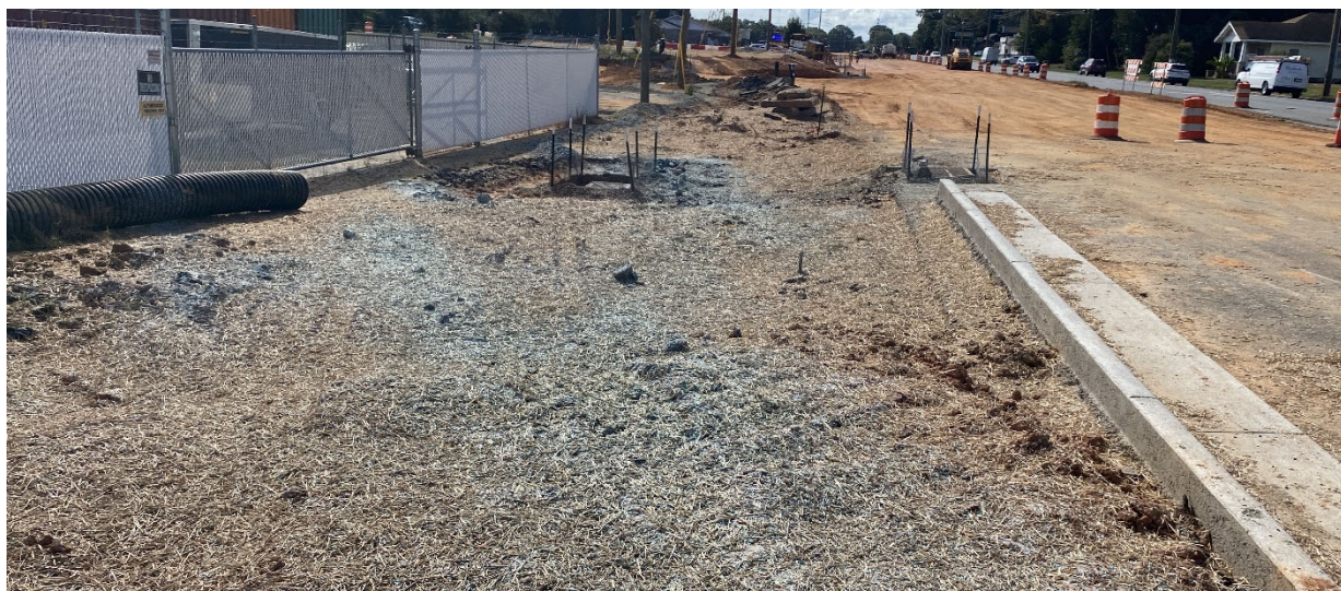
Drop Inlet Protection measures.
