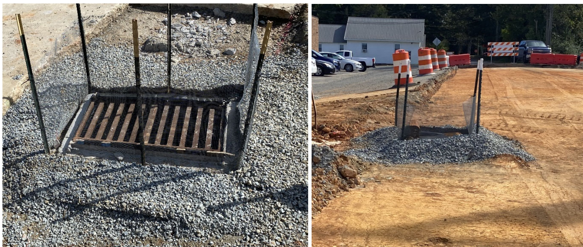
Drop Inlet Protection measures.
