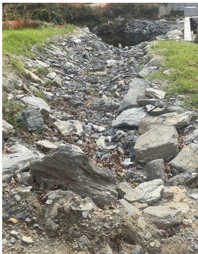
Completed permanent ditch and stabilized stream bank.
