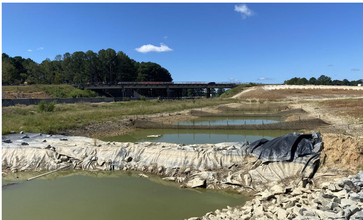
Additional skimmer basin installed and holding water.
