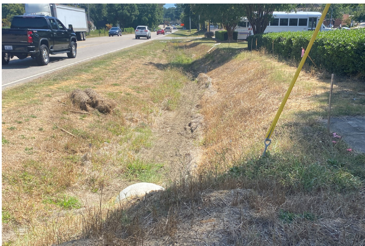
Completed ditches stabilized.
