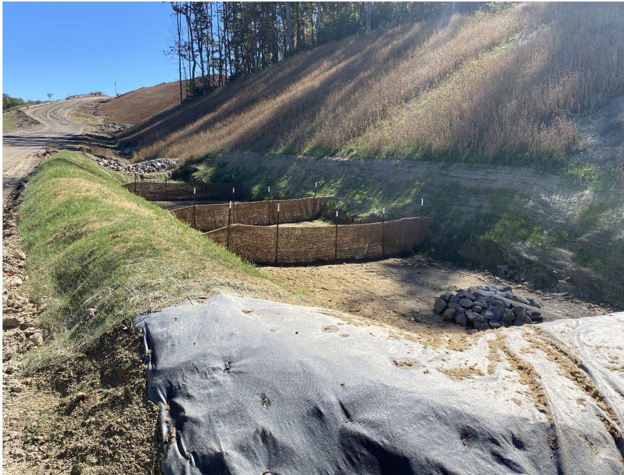
Skimmer basin and adjacent slopes that had been stabilized.
