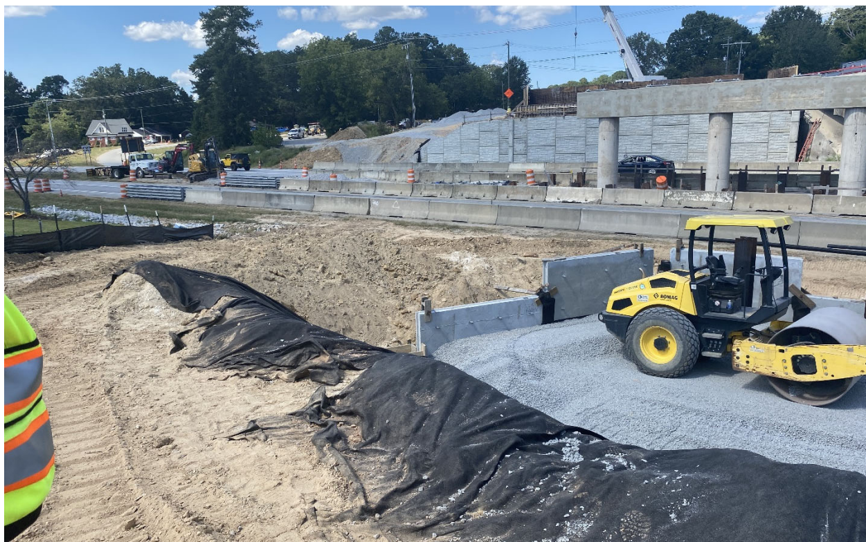
Bridge construction underway.
