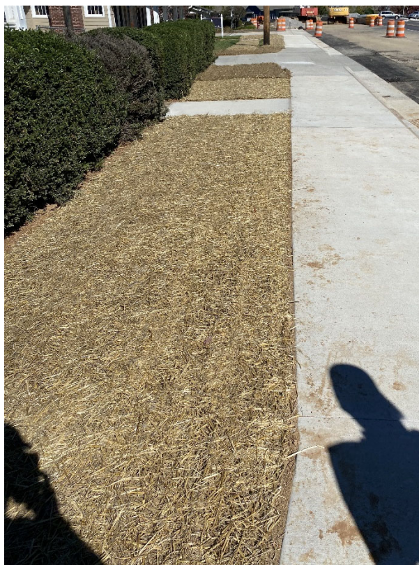
Completed areas seeded and mulched with straw or matted.
