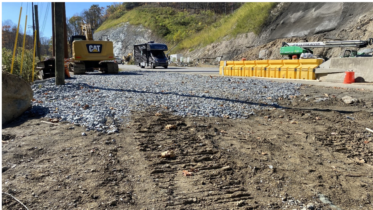
Construction entrance is maintained.
