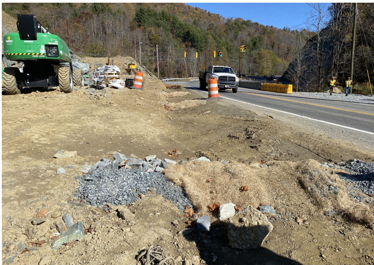
Check dams installed or recently maintained.
