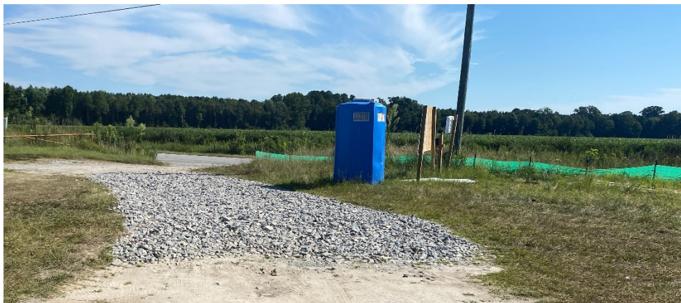
Construction Entrance to Staging Area
