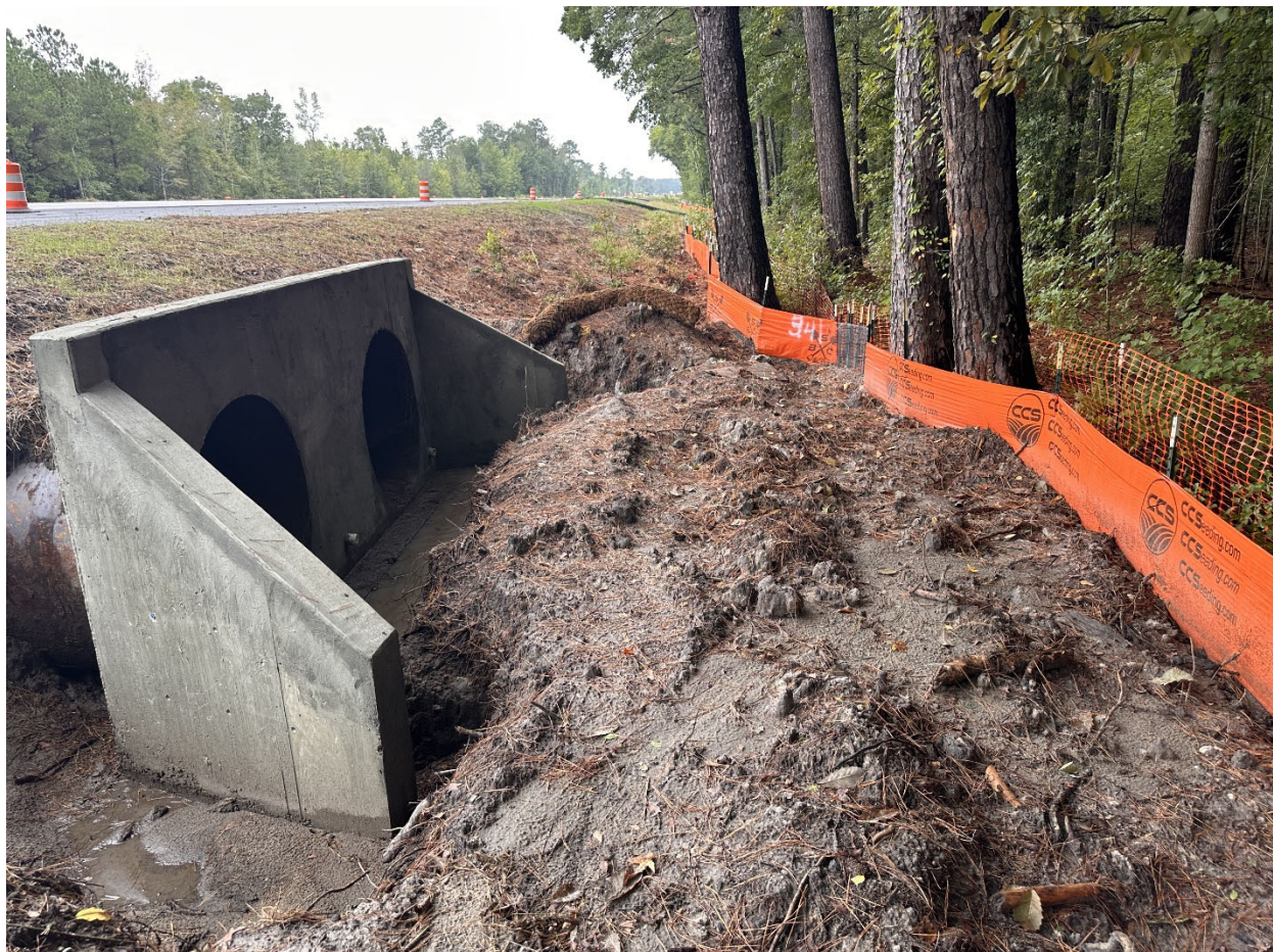
Culvert extension installed.
