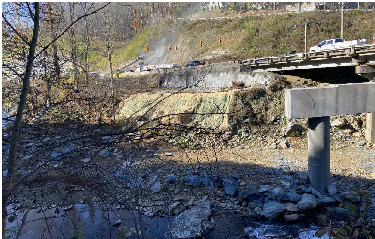
Slopes matted below new bridge approach.
