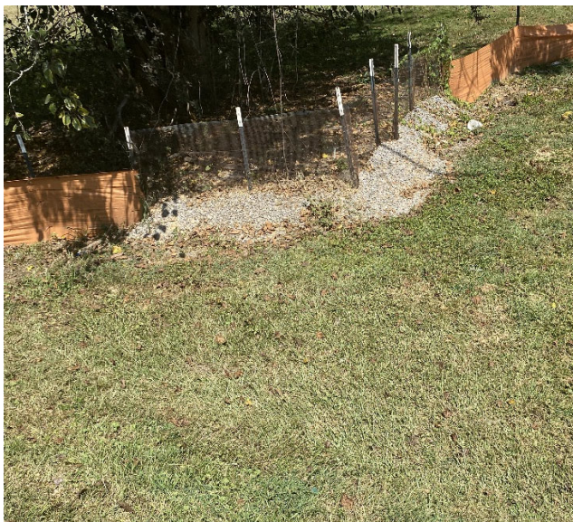
Silt fence outlets and check dams.
