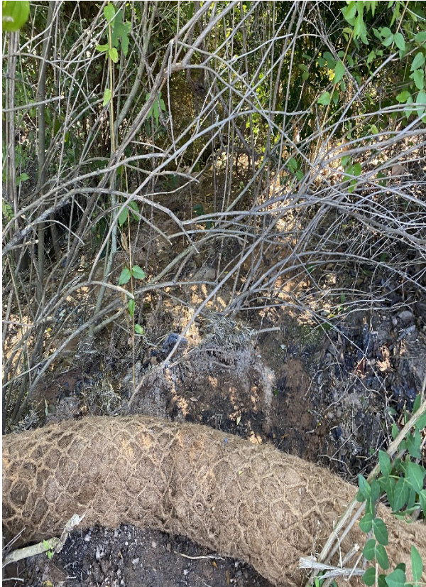
Minor sediment loss needing to be retrieved and additional measures added around flume.
