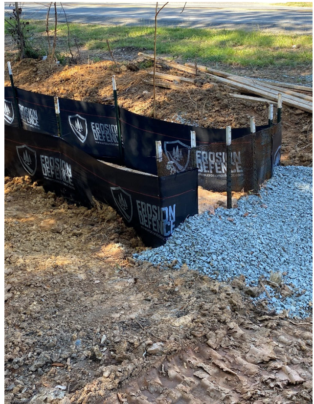
Minor sediment loss needing to be retrieved and additional measures added around flume.
