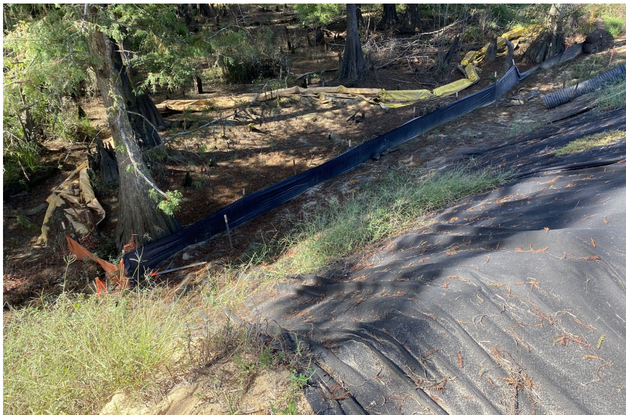
Turbidity curtain added to address high-water levels.
