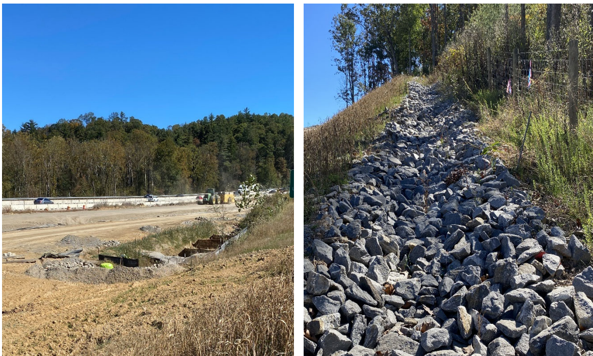
Additional Skimmer Basin installed and Clean Water Diversion
