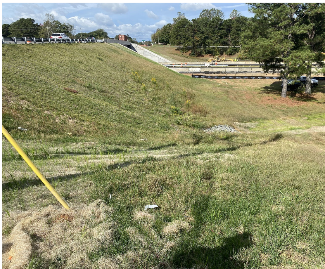
Slope completed and stabilized.
