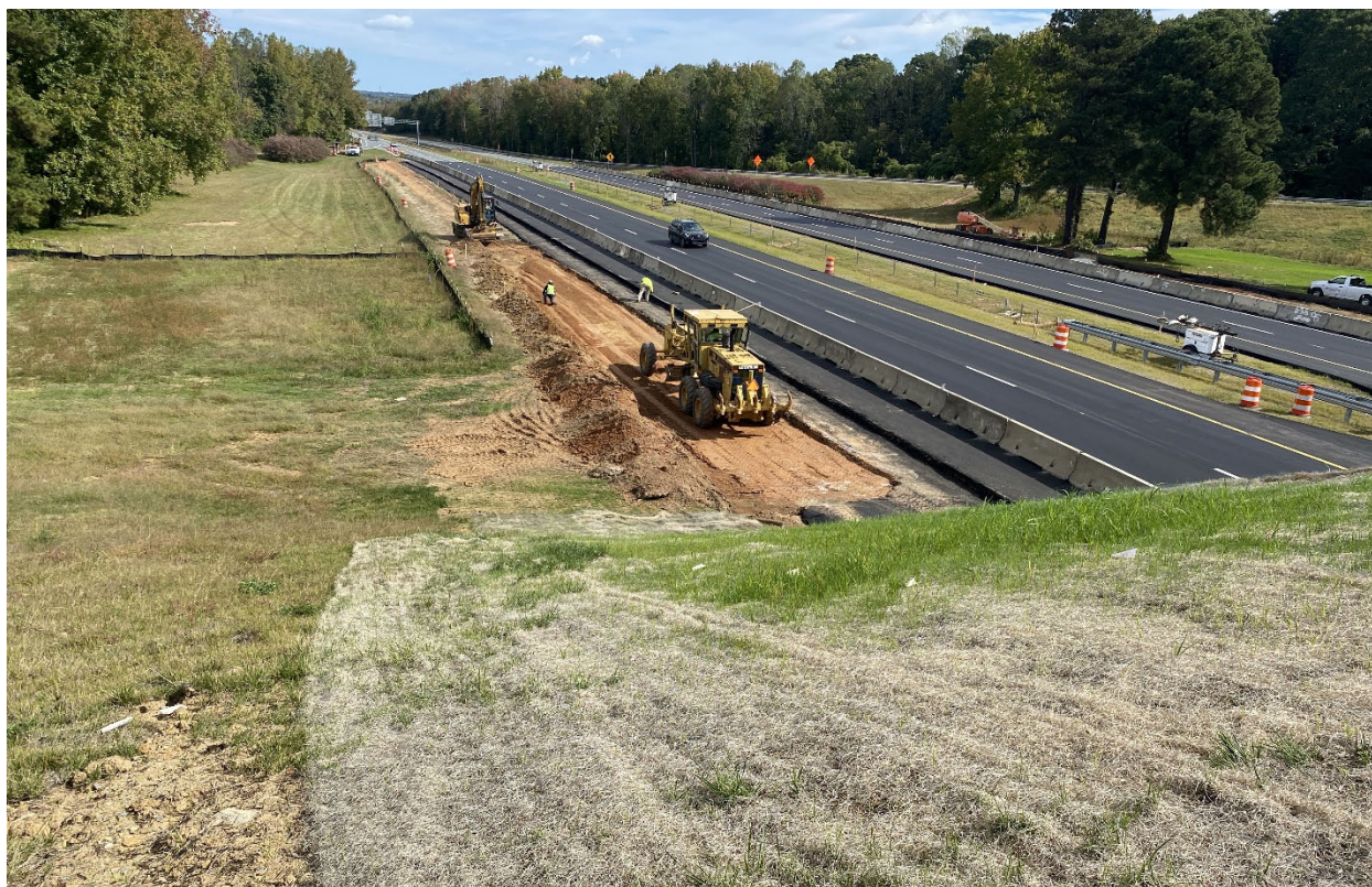
Grading for widening underway.
