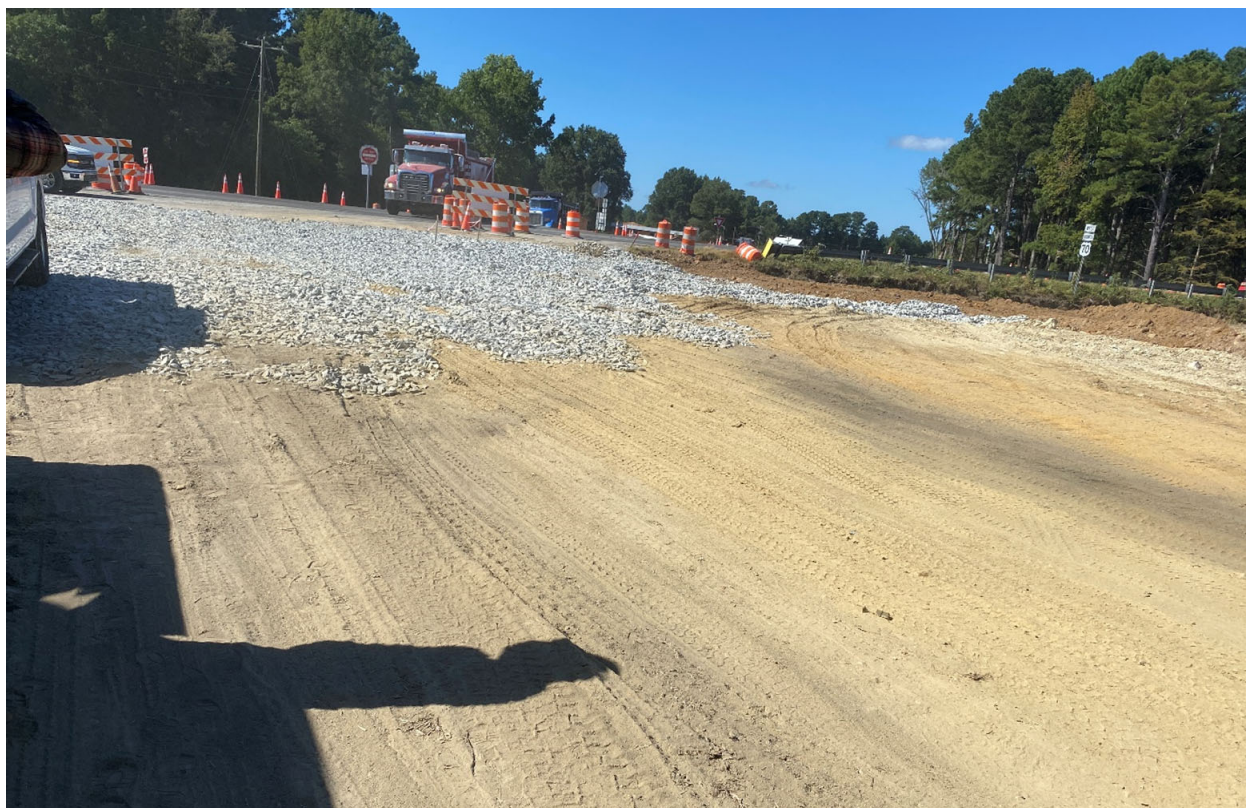
Construction entrance installed.
