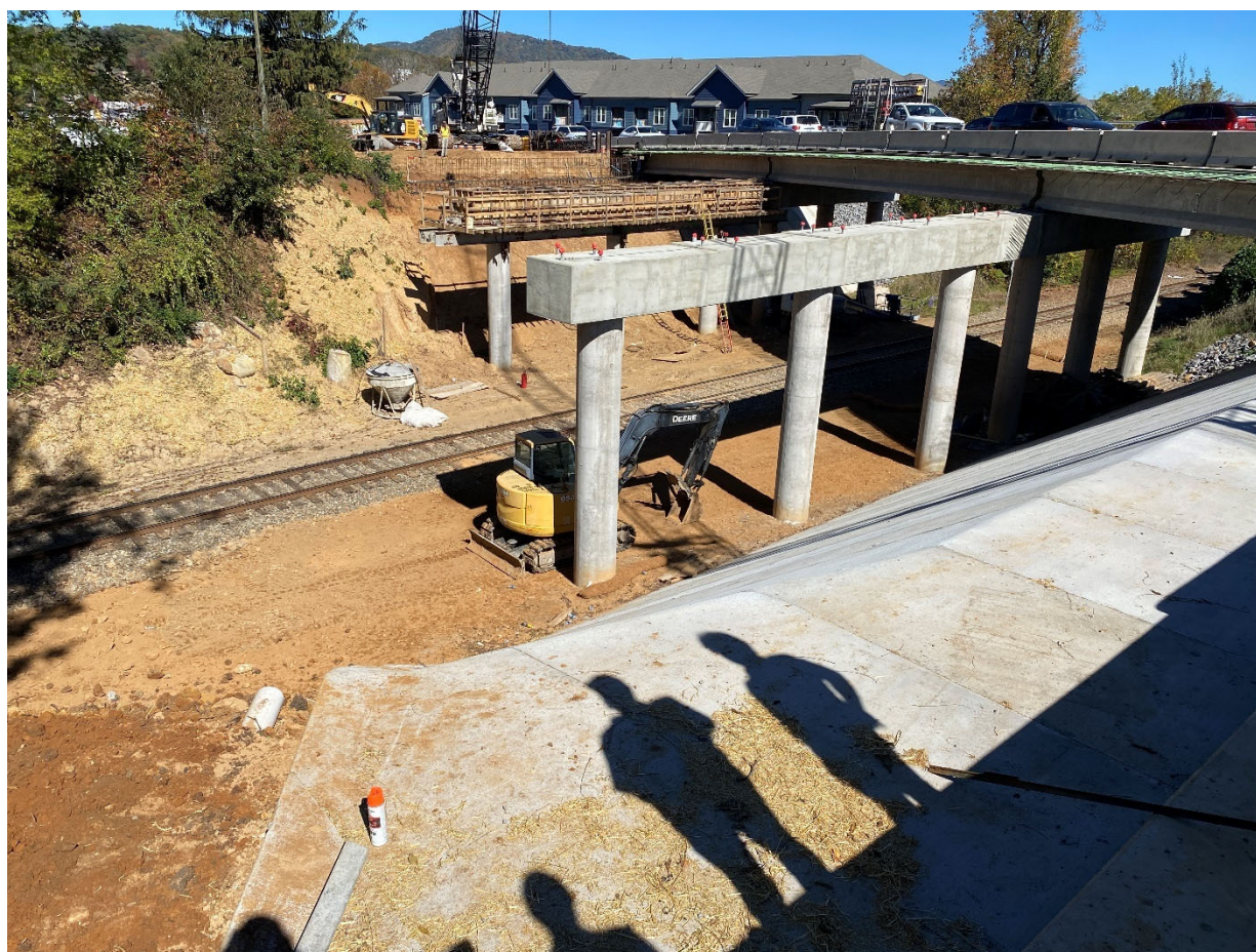
Bridge construction underway.
