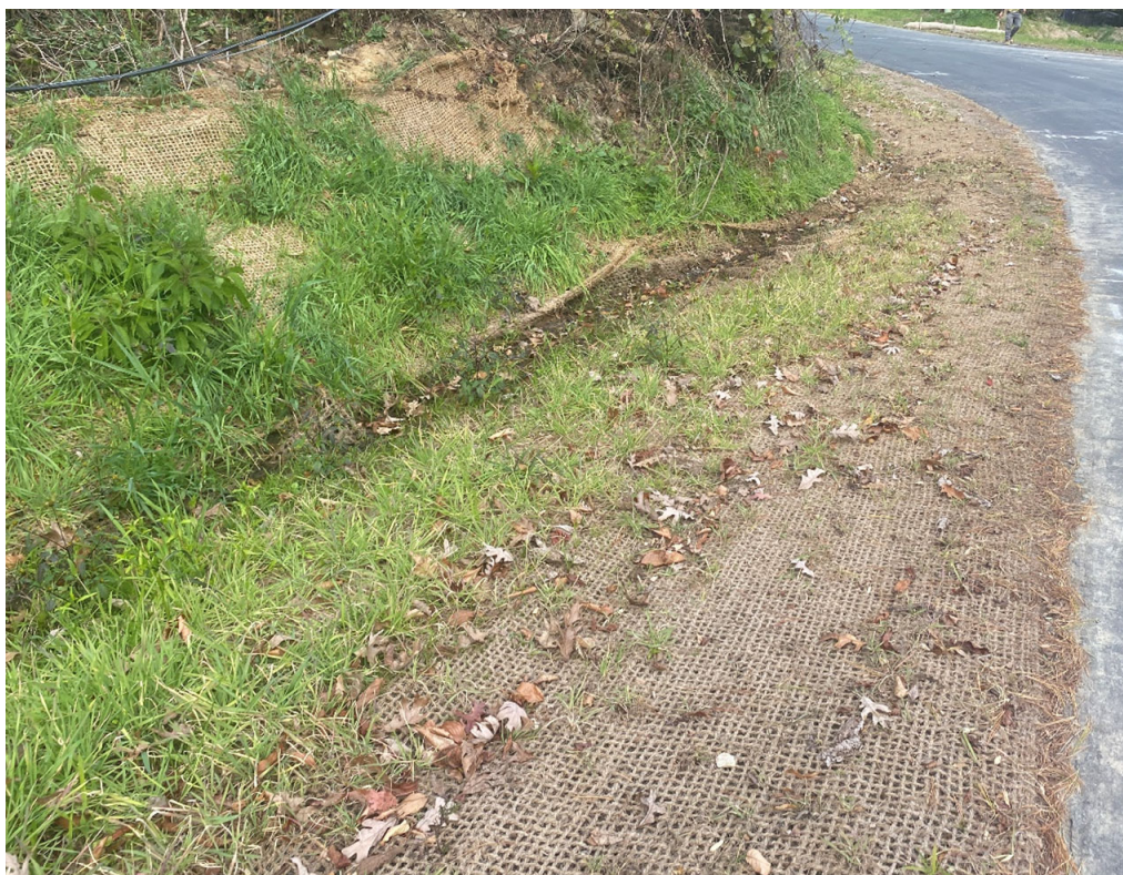
Roadside ditch being stabilized.
