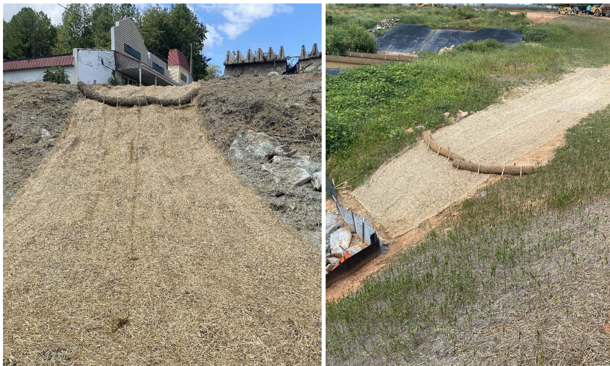
Rill repairs completed.
