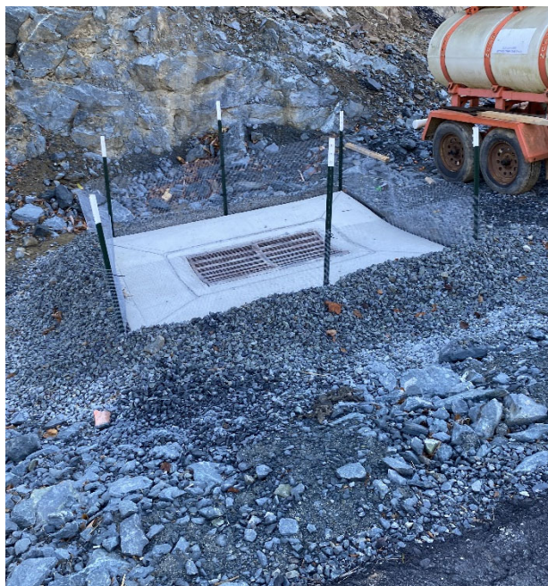
Drop inlet protection measures installed.
