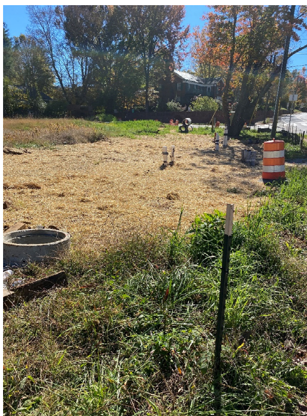
Completed areas seeded and mulched with straw or matted.
