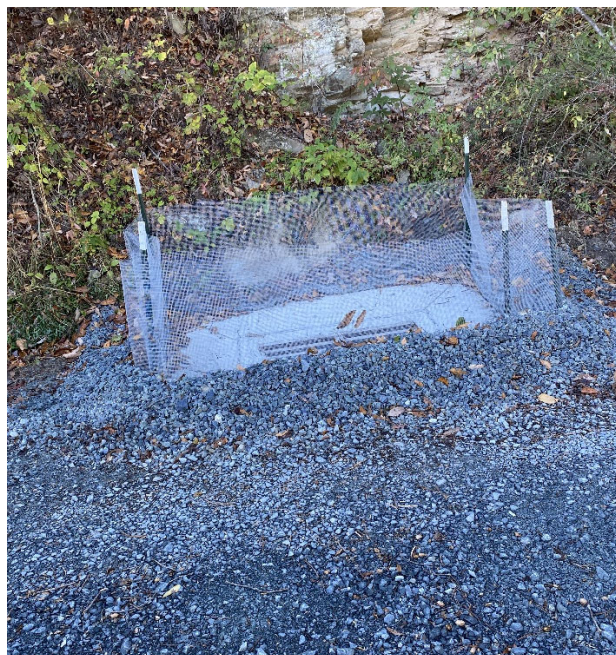
Drop inlet protection measures installed.
