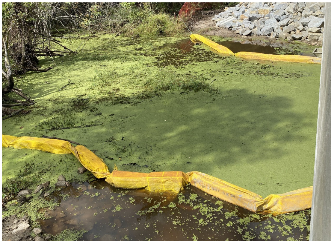
Turbidity curtains installed.
