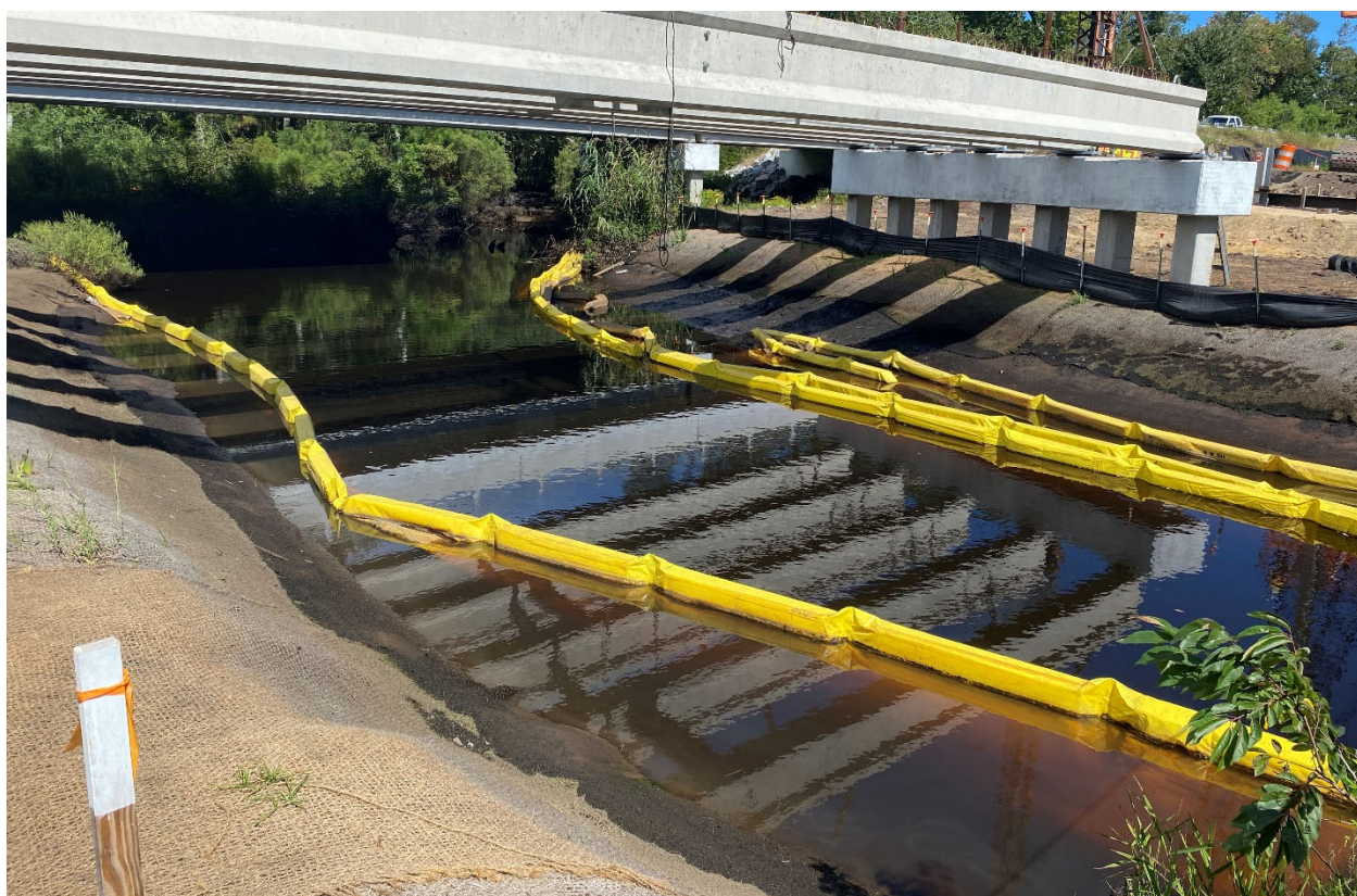
Special Sediment Control Fence, Wattles and Turbidity Curtains installed at bridge construction.
