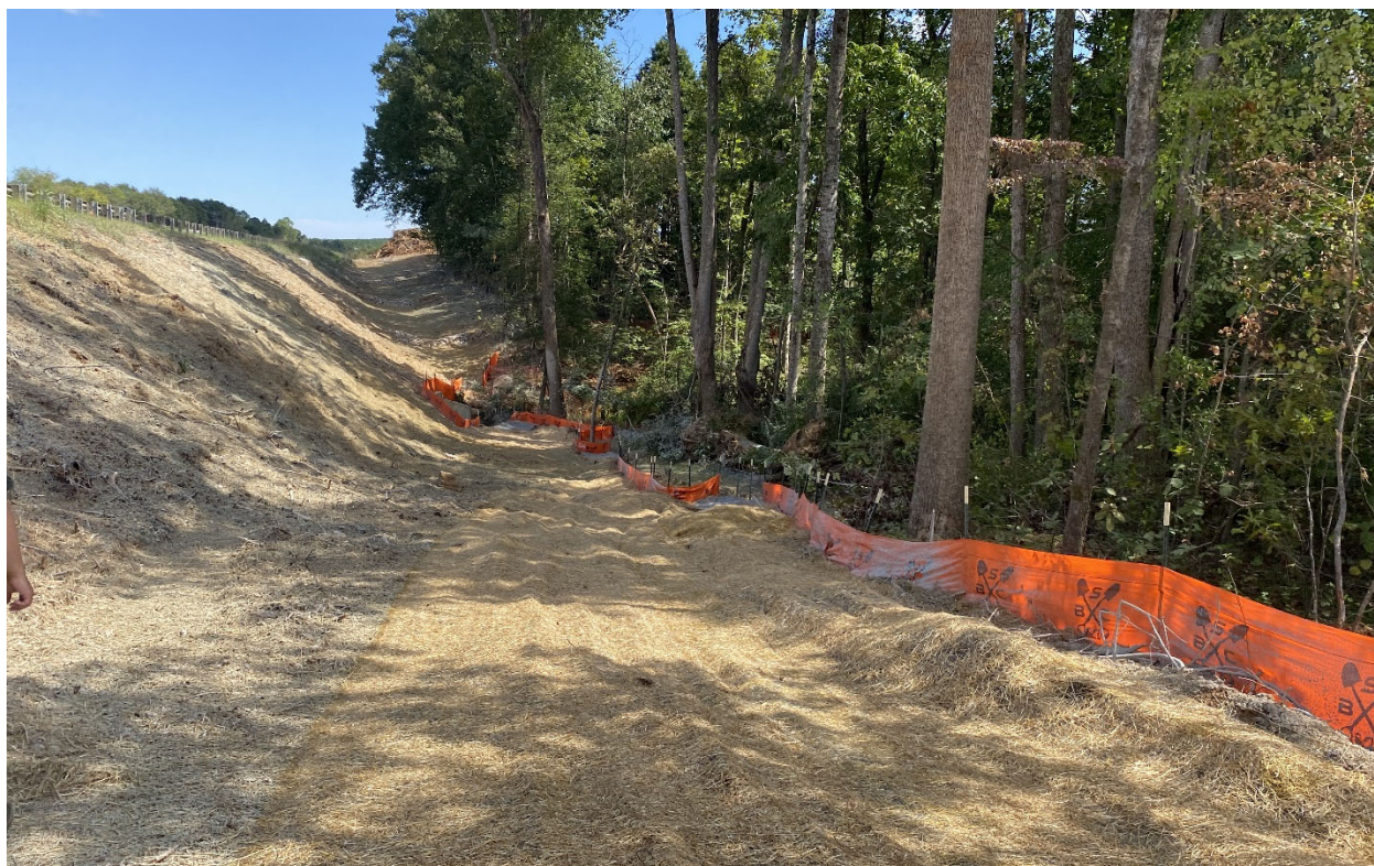
Completed slopes being stabilized.
