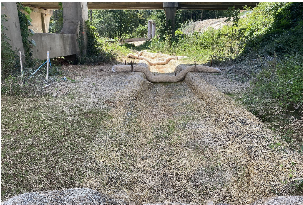
Diversion ditch installed with wattles below bridge.
