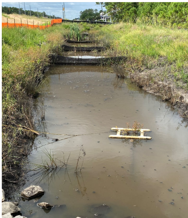
Skimmer Basins installed and maintained.
