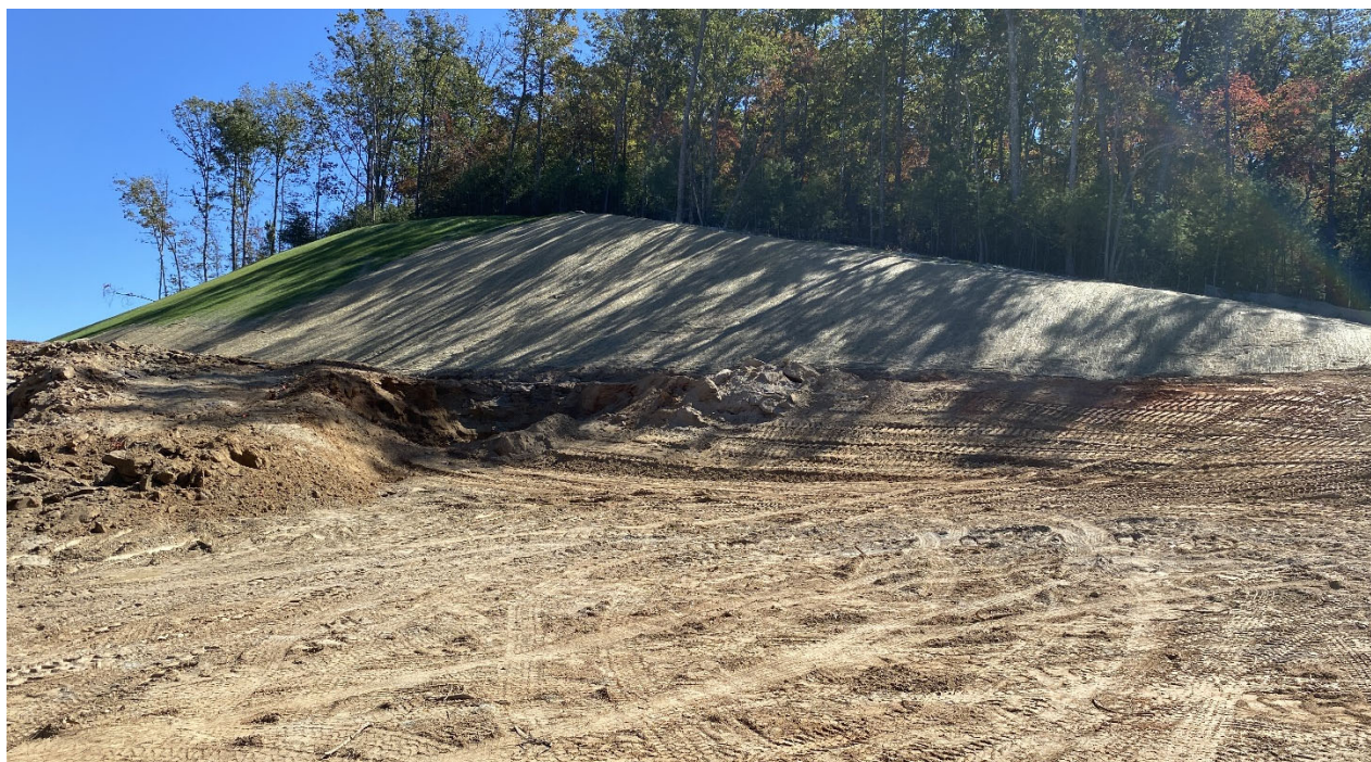
Slopes being stabilized.
