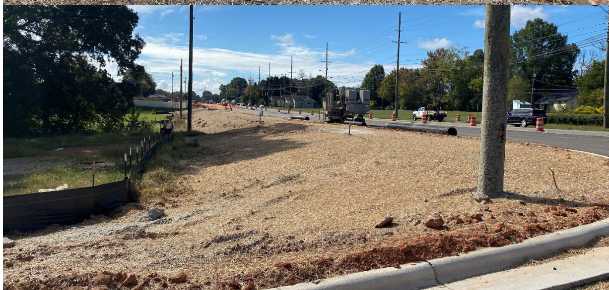
Disturbed Areas seeded and mulched with straw.
