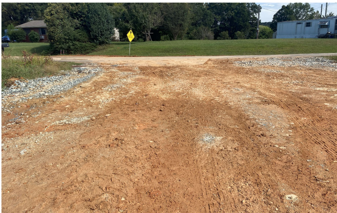
Borrow/waste site construction entrance.
