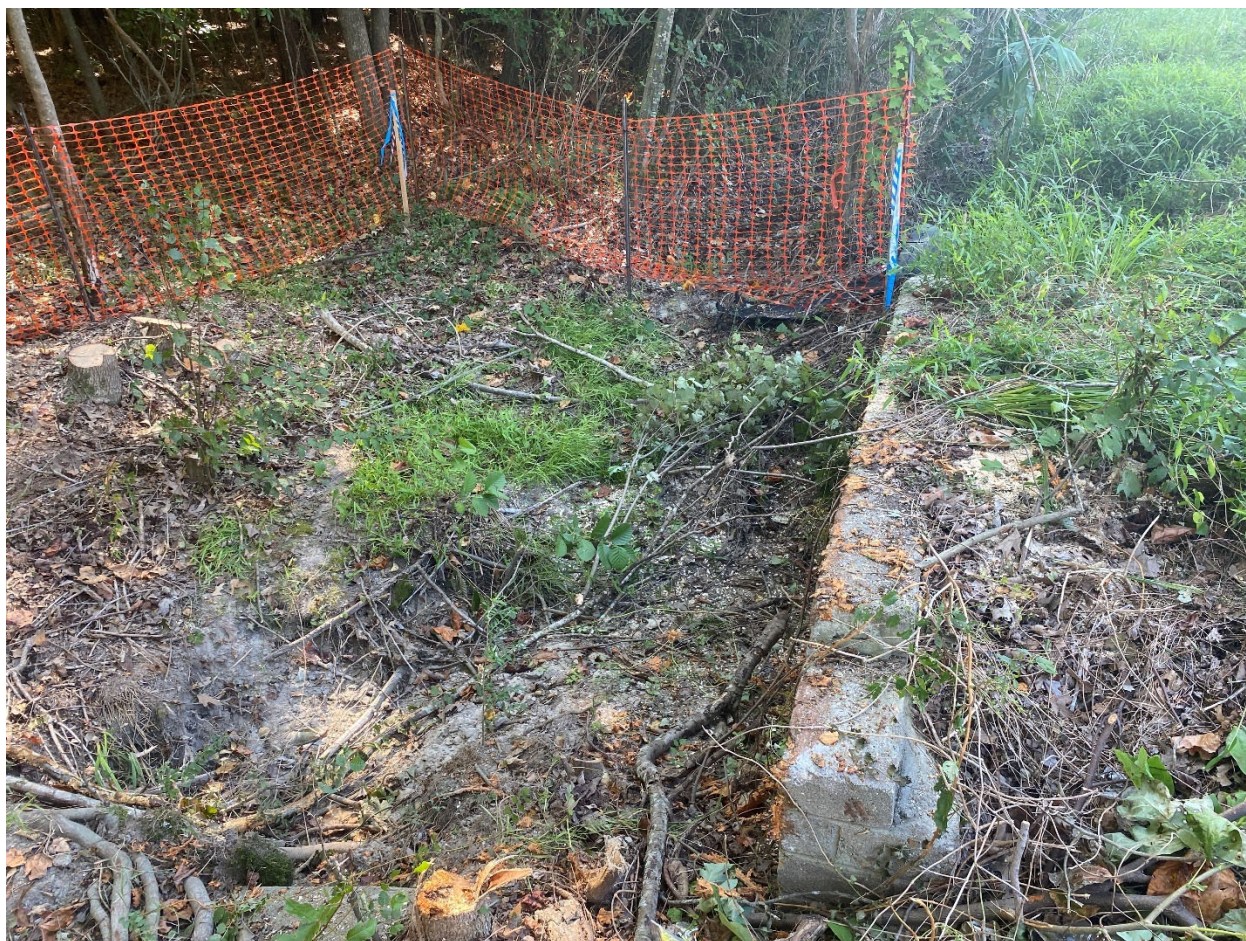
Safety fence installed and clearing began
