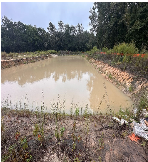
Stilling basins at the borrow pits would need to be repaired before any future use.
