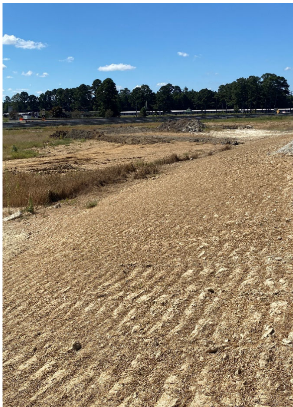
Slopes mulched with straw and hydro mulch
