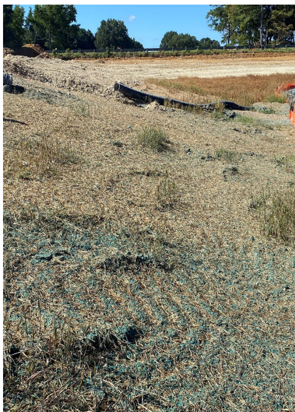
Slopes mulched with straw and hydro mulch
