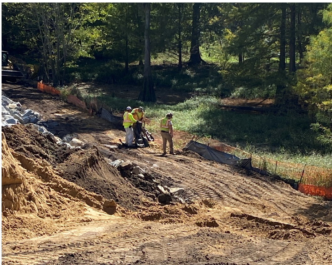
Silt fence repairs started.
