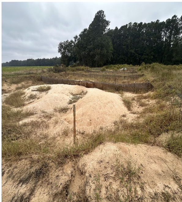
Stilling basins at the borrow pits would need to be repaired before any future use.
