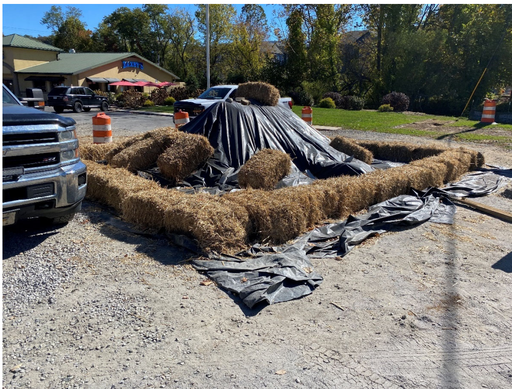
Contaminated soils storage.
