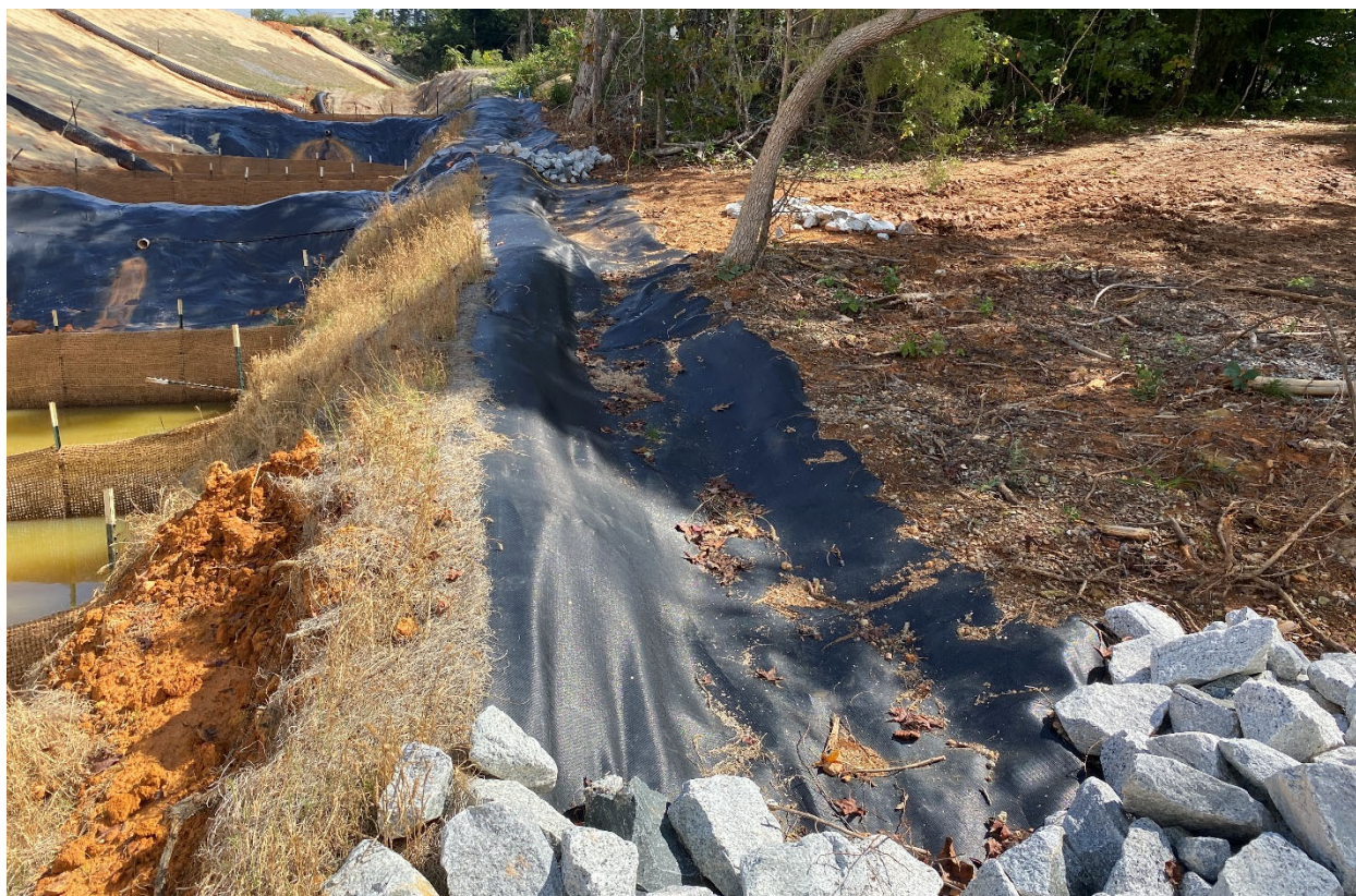
Clean water diversion installed.
