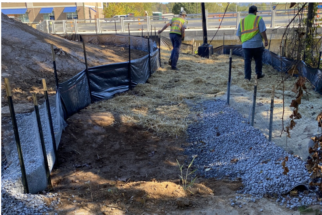
Perimeter measures around staging area.
