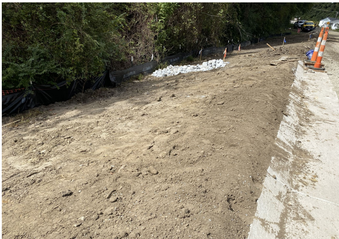
Slopes being fine graded nearing completion.
