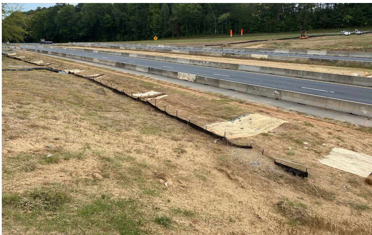
Check dams and wattles installed.
