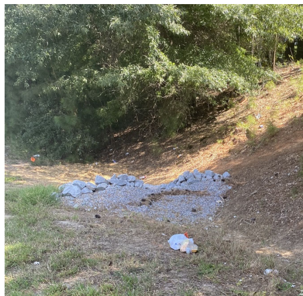
Silt fence outlets and check dams.
