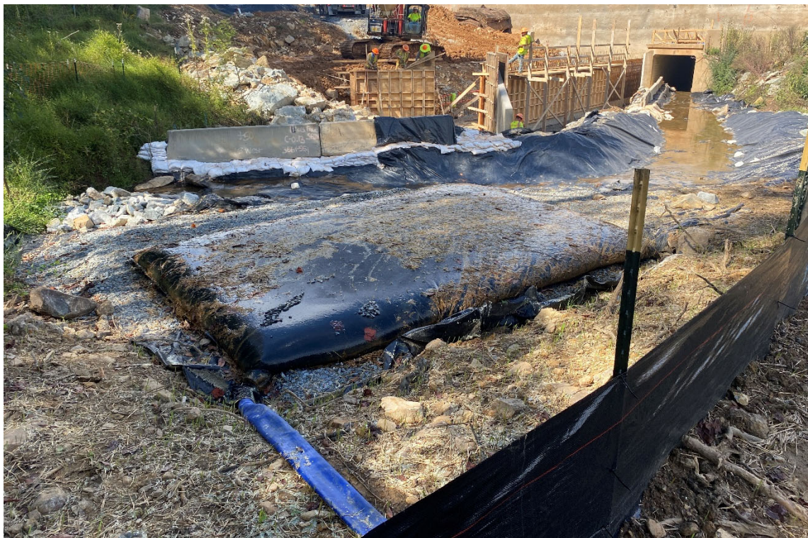
Silt bag for dewatering culvert installation work area.
