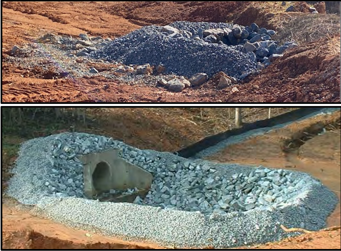
Figure 6.55b, Examples of Rock Pipe Inlet Protection
