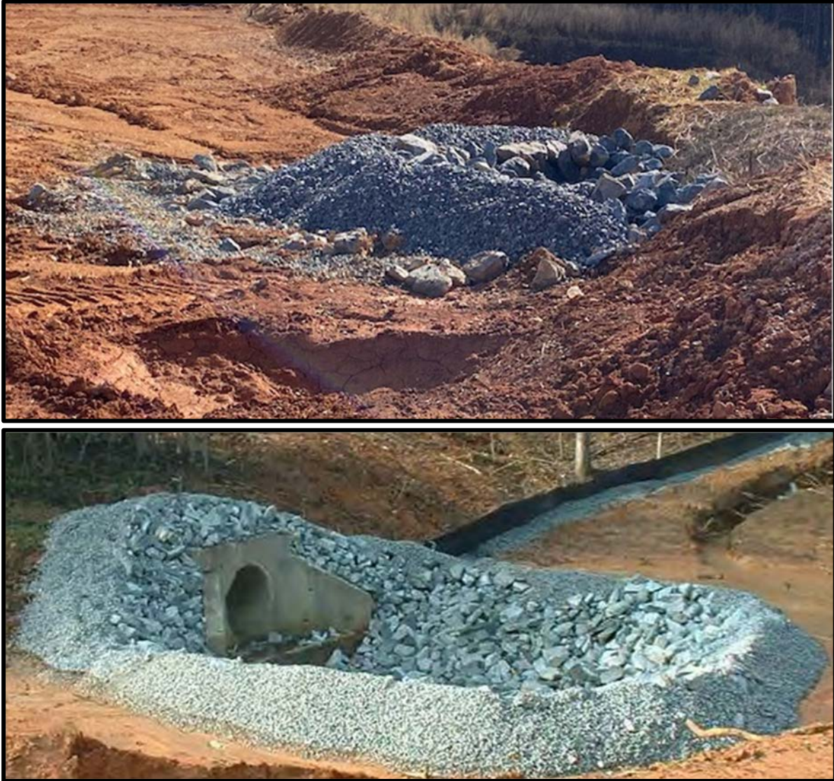
Figure 6.55b, Examples of Rock Pipe Inlet Protection
