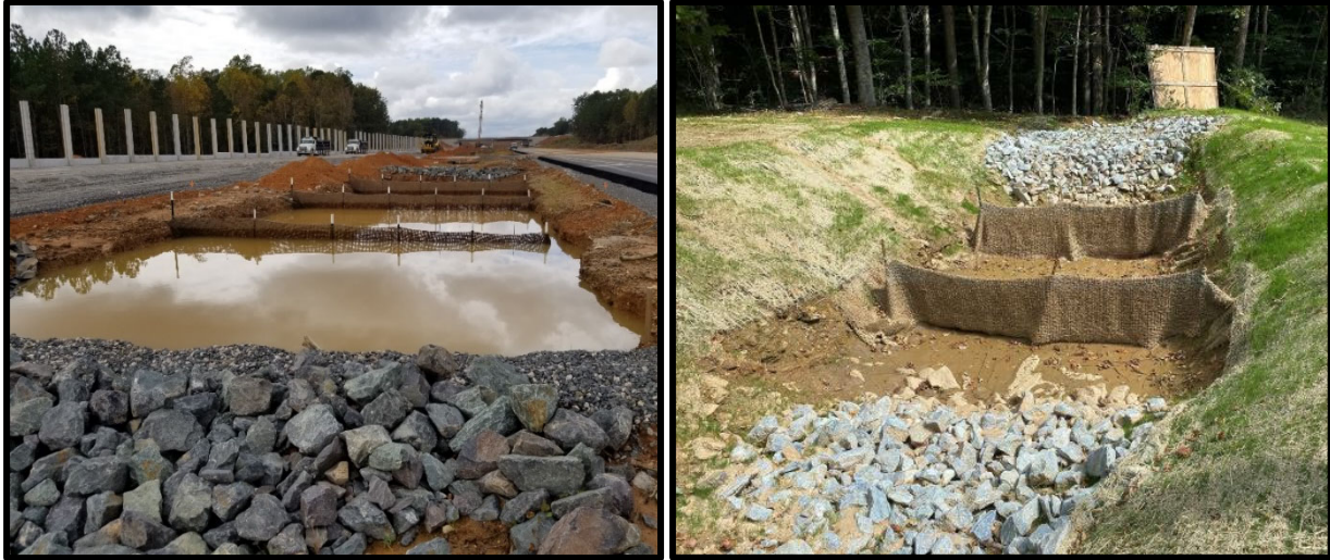
Figure 6.60b Temporary Sediment Trap collects runoff to allow sediment to settle.
