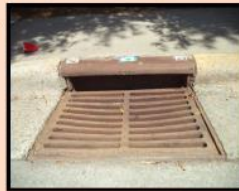
Drainage systems are designed to reduce localized flooding. Storm drains discharge to ditches, streams and lakes without treatment.
