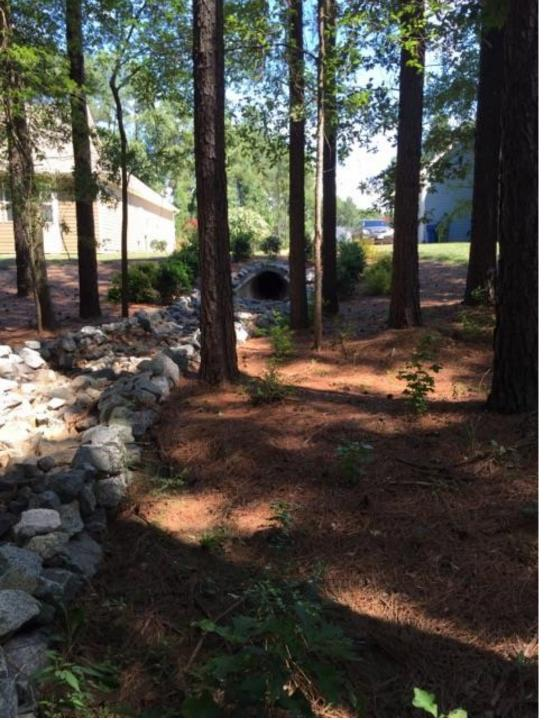
Stormwater discharge from public right of way infrastructure includes a plunge pool and rip rap swales to dissipate velocity, spread flow, and minimize or eliminate erosion
