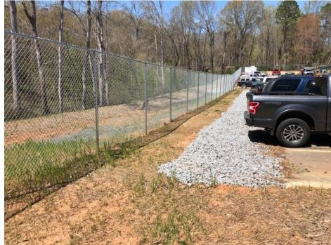
The PW Facility used a combination of an infiltration trench and a level spreader
