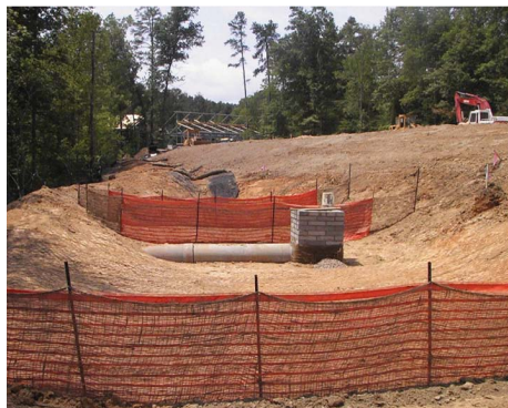
Figure 1. Skimmer basin now converted to constructed wetland with a bottom outlet (see stone at bottom of riser). Note inlet protection and wattles on the ditch at the far end.
