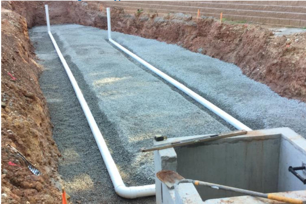
Figure 4: Typical Bioretention Underdrain
