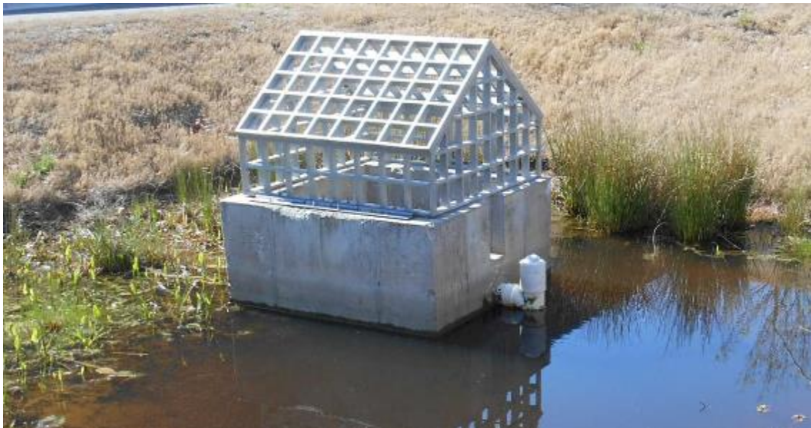
Figure 7: Typical Trash Rack
