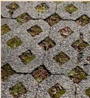
CGPs are an “older cousin” to PICPs and have significantly larger openings filled with aggregates, sand, or topsoil and turf grass for infiltration. CGPs are intended for limited vehicular traffic such as overflow parking (e.g., intermittent stadium parking), emergency access fire lanes around buildings, and median crossovers. CGP is not recommended for regularly used parking areas and for roads intended for PICP or PC.
