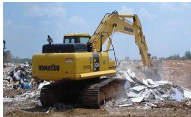
Making up approximately 5 percent of the total C&D recovery, drywall (shown above) is separated and processed for recycling at various sites across the state.
