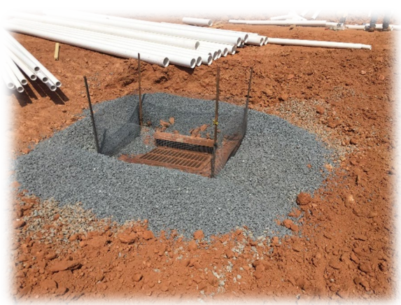
Figure 12 - Good Inlet Protection
