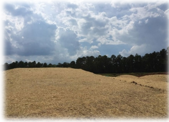
Figure 8 - Good Application of Ground Cover
