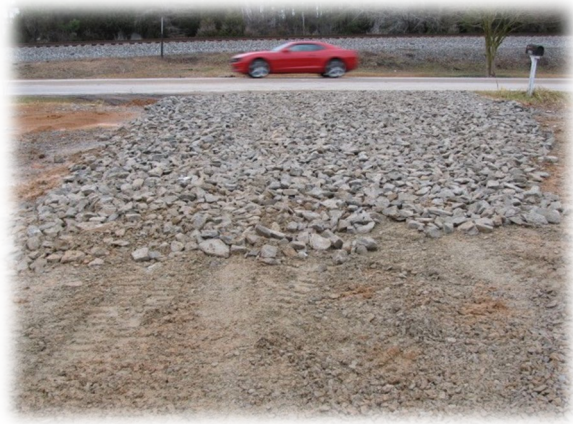
Figure 6 - Good Construction Entrance
