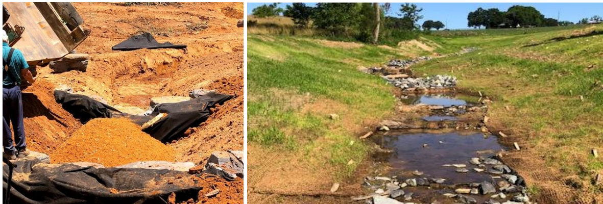
Figure 3. Section of NT stream RSC during construction (left) and after completion (right)
