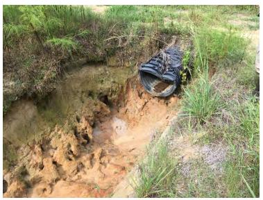
UT3: Severe erosion in northwest corner.
