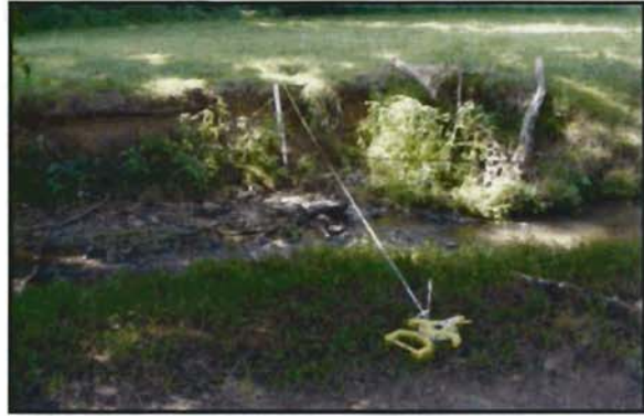
8-4 right bank looking left bank
