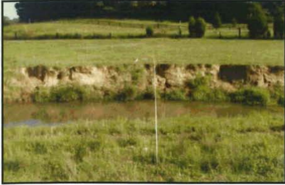
8-2 left bank looking right bank
