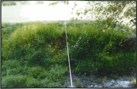
8-5 left bank looking right bank
