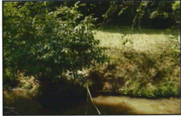
8-3 right bank looking left bank
