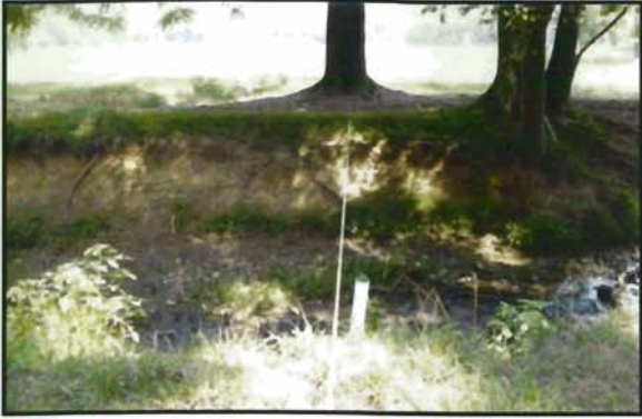
8-4 left bank looking right bank
