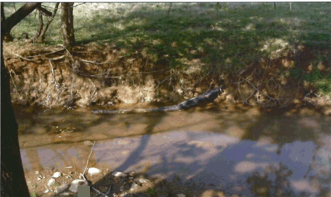
**Photograph 4 – Three-inch (3") drain enters the stream from the west bank at Station 10+80.**
