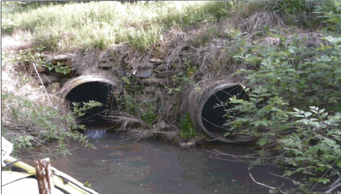
Photograph 1 – Two 36" RCPs mark the upstream extent of the project reach (Station 10+00, looking upstream).
