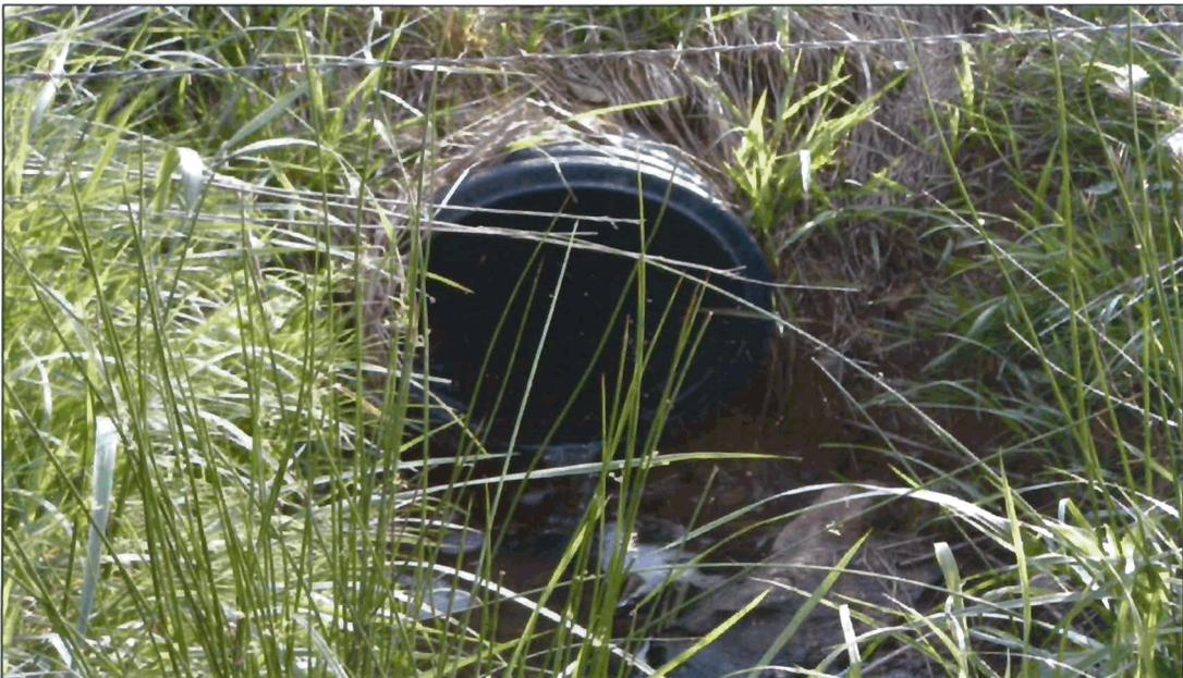
**Photograph 12 – A 12” plastic pipe that serves as the overflow drain from the pond enters the left bank of UTJC2 at Station 54+93.**
