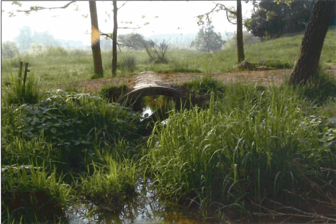
Photograph 7 – Thirty-six inch (36") RCP serves as the primary stream crossing on UTJC2. The structure is located from Station 52+17 to 52+31.
