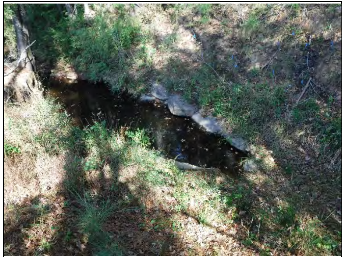
PP-22: Reach UT4-R3 – View downstream, Station 31+00
