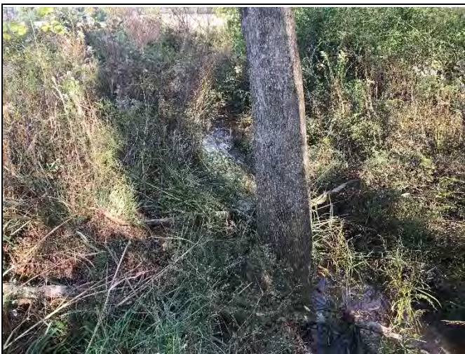
PP-23: HC Reach 3, view downstream at Station 15+50
