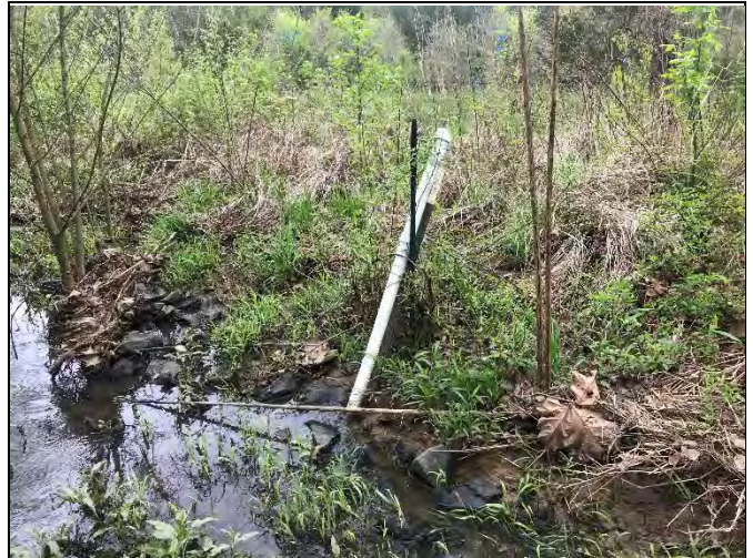
Flow Gauge in upper Reach HC-R1 (photo 4/12/19)
