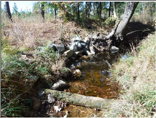
PP-19: Reach UT4-R3 – View downstream, Station 29+00
