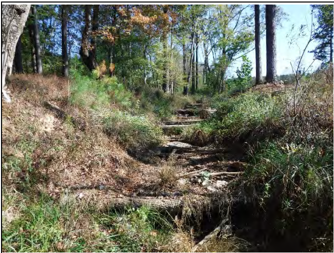
PP-23: Reach UT4-R2 – View upstream at Station 37+50
