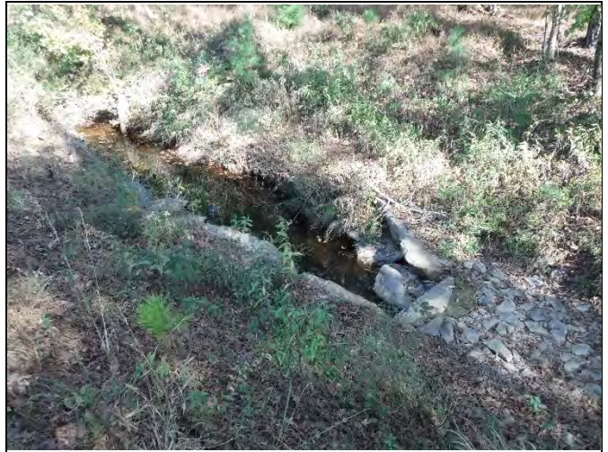
PP-20: Reach UT4-R3 – View downstream, Station 29+50
