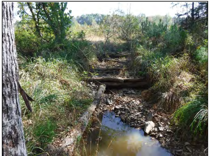
PP-24: Reach UT4-R2 – View upstream, Station 37+00
