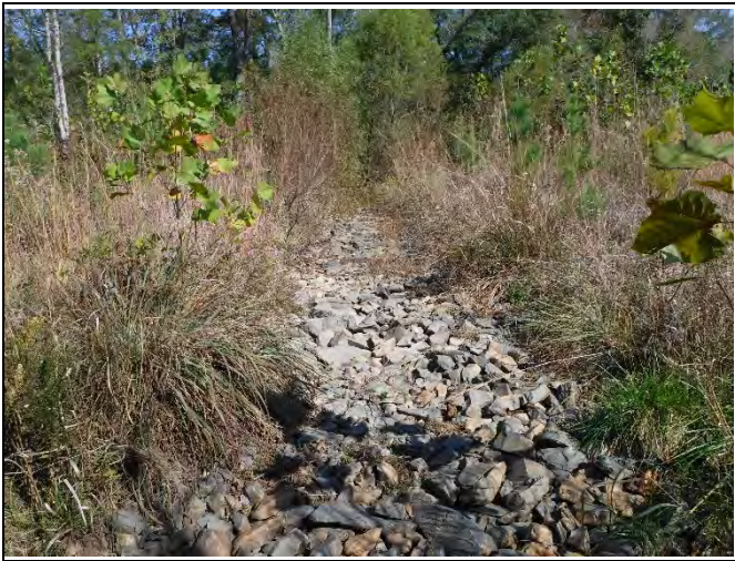
PP-27: Reach UT4-R2 – View upstream, Station 31+50
