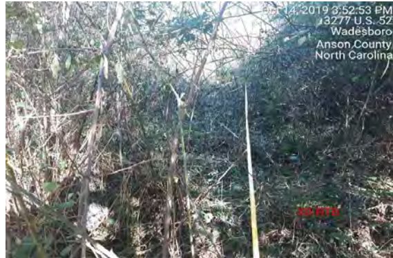
Looking at the Right Bank
