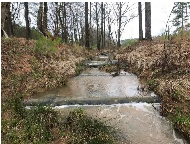
PP-23: Reach UT4-R2 – View upstream at Station 37+50
