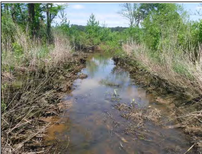
PP-11: HC Reach 1, view downstream at Station 29+30
