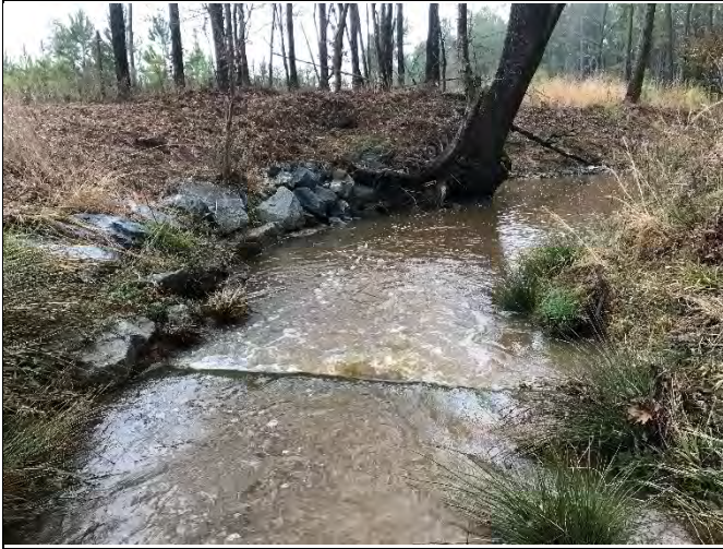
PP-19: Reach UT4-R3 – View downstream, Station 29+00
