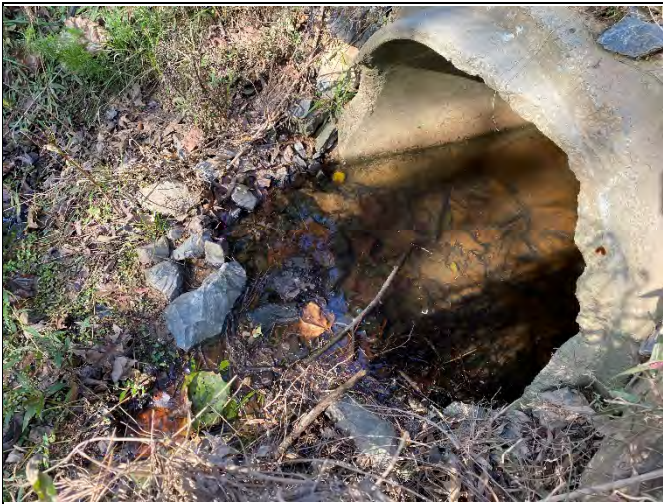
Pipe under crossing at UT4-R1a and R1b
