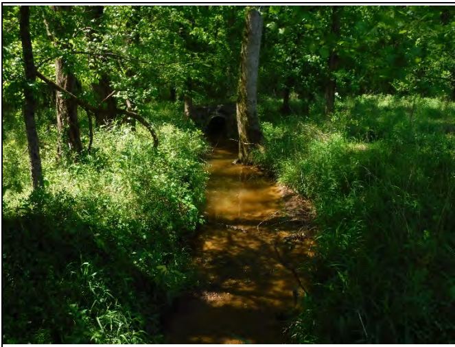
PP-21: HC Reach 3, view upstream at Station 11+40
