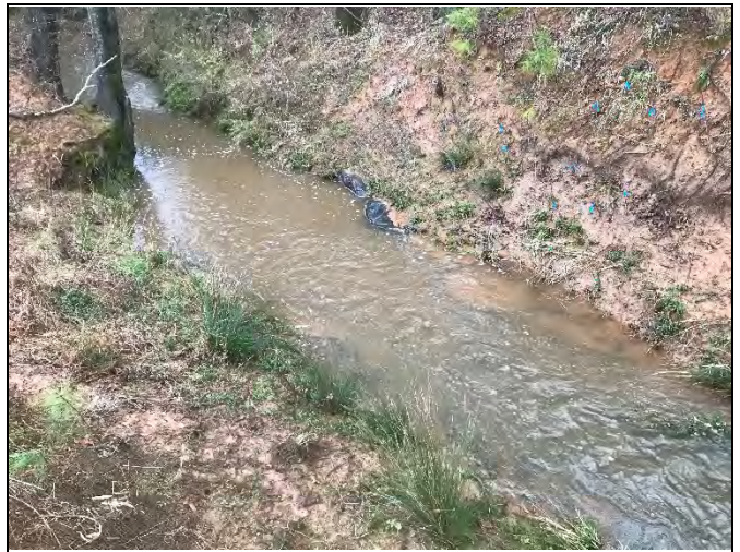
PP-22: Reach UT4-R3 – View downstream, Station 31+00
