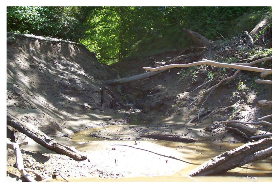
Location:Confluence of the Deep River and an unnamed tributary near Monitoring Station 23Description:Severe headcutting and erosion of bank material
