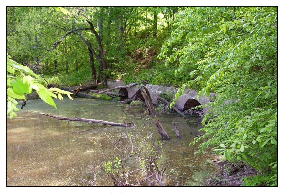
Location:Upstream of Carbonton Road and Line Creek crossingDescription:Coarse woody debris at culvert intake leading under Carbonton Road
