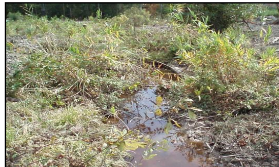
Sod mats blanket the top of bank of this stream in Bertie County.
