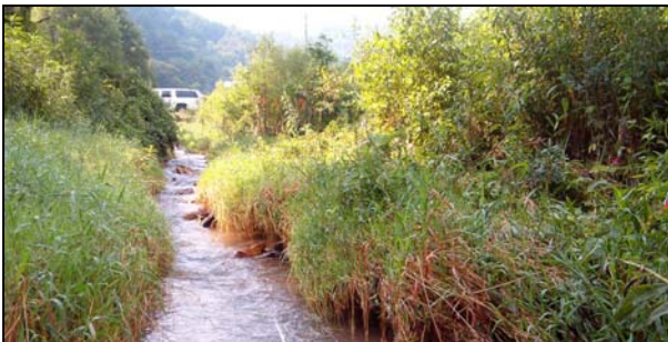
Facing upstream at undercut banks at Station 5+65 - June 2004
