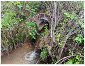
drop at the pipe outlet into the pool planned downstream, but that aquatic connectivity remains an unlikely result of this work under the circumstances. The change will help protect the pipe from undermining any further and may provide the possibility of passage under some circumstances. This change has been made to the plans.
