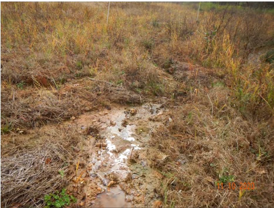
SPA5, R5 Left Floodplain, Minor Erosion (MY-01)
