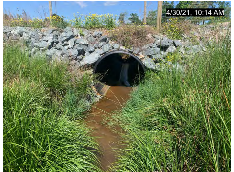
PS-1, R1, Culvert Crossing, Upstream (MY-02)
