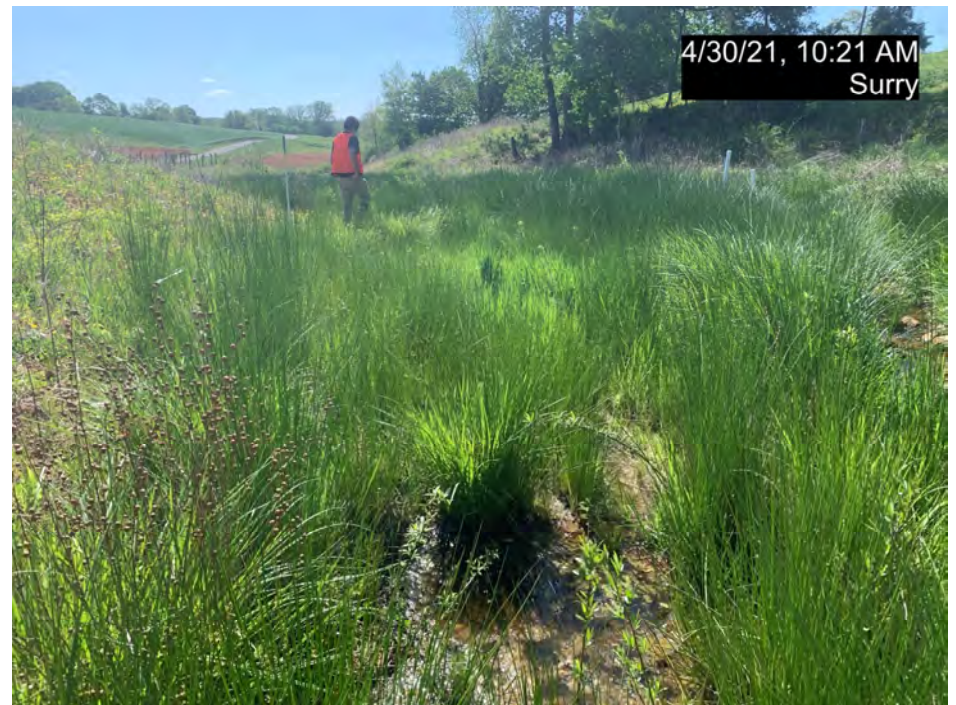
SPA3, R1 Left Floodplain, Minor Erosion (MY-02)
