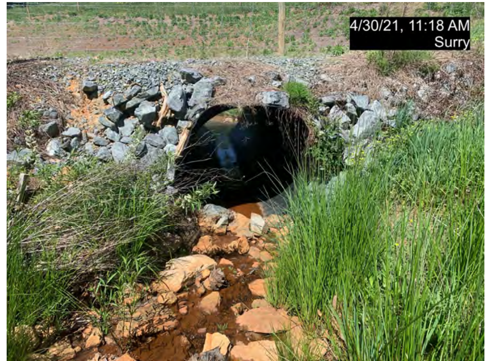
PS-2, R2, Culvert Crossing, Downstream (MY-02)
