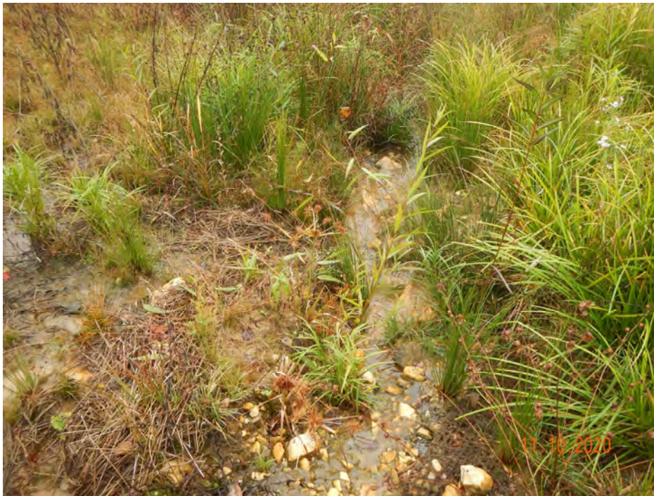
SPA3, R1 Left Floodplain, Minor Erosion (MY-01)
