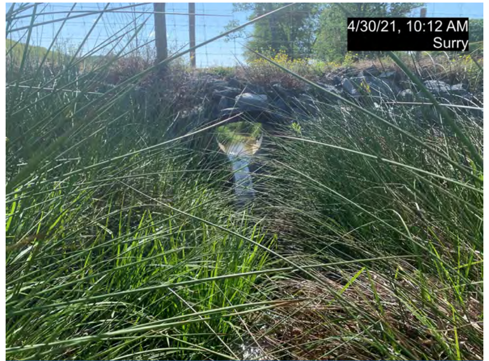
PS-1, R1, Culvert Crossing, Downstream (MY-02)
