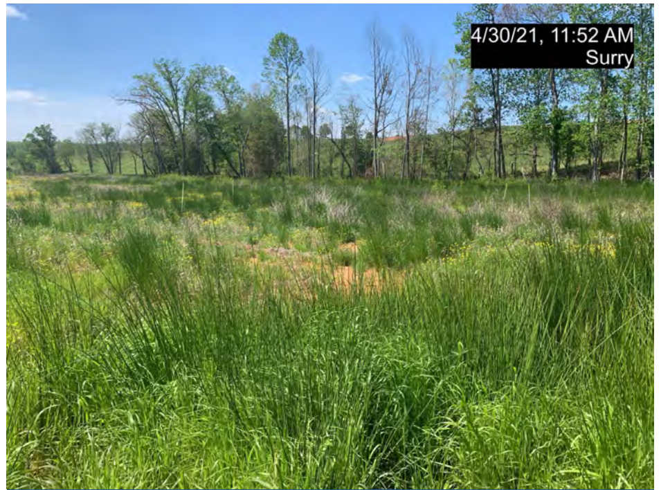
SPA5, R5 Left Floodplain, Minor Erosion (MY-02)
