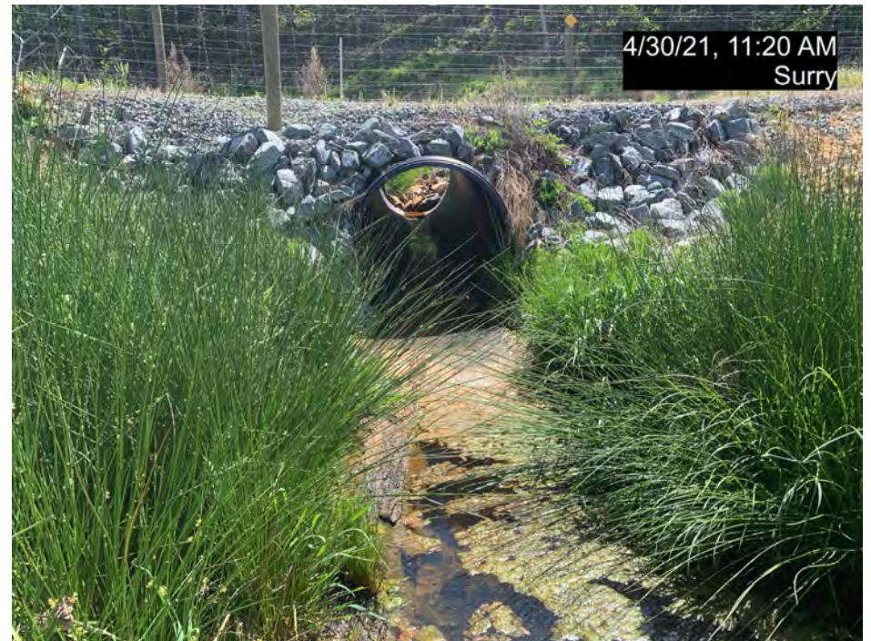
PS-2, R2, Culvert Crossing, Upstream (MY-02)
