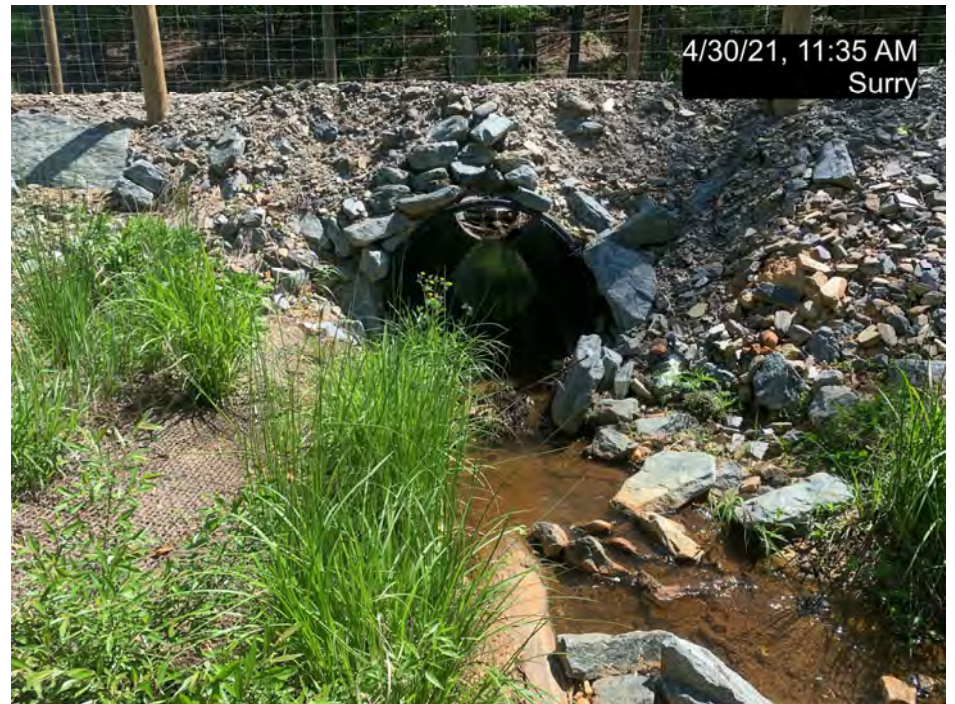
PS-3, R4, Culvert Crossing, Upstream (MY-02)
