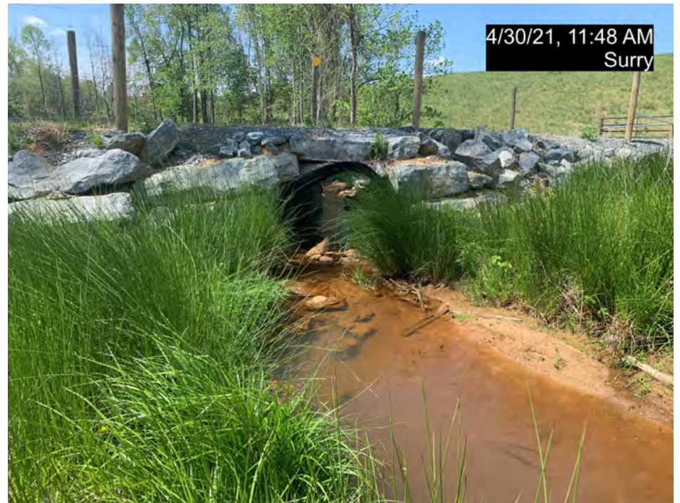
PS-6, R5, Culvert Crossing, Downstream (MY-02)
