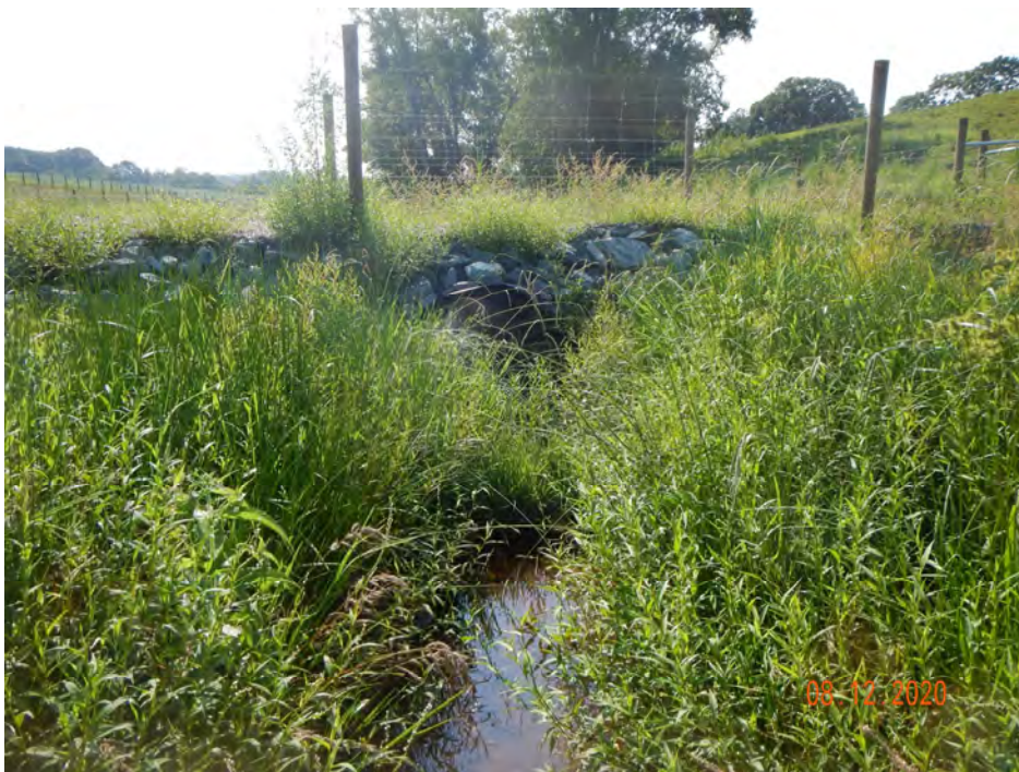
PS-1, R1, Culvert Crossing, Downstream (MY-00)
