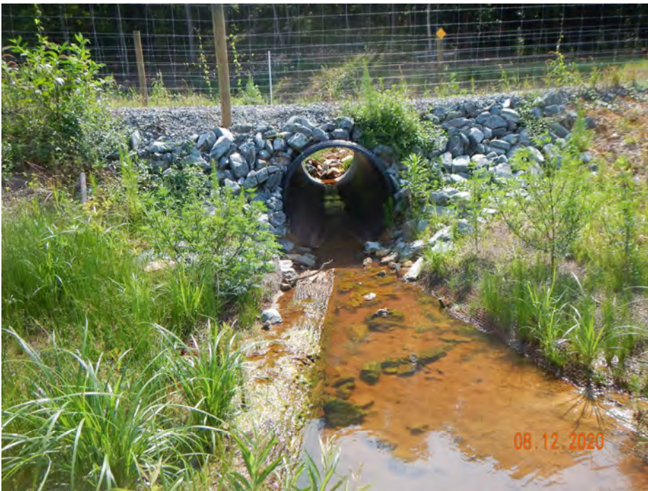
PS-2, R2 Culvert Crossing, Upstream (MY-00)
