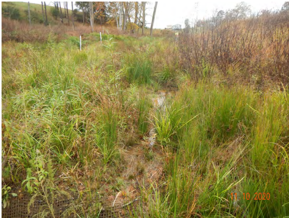
SPA3, R1 Left Floodplain, Minor Erosion (MY-01)
