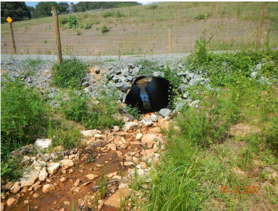
PS-2, R2, Culvert Crossing, Downstream (MY-00)
