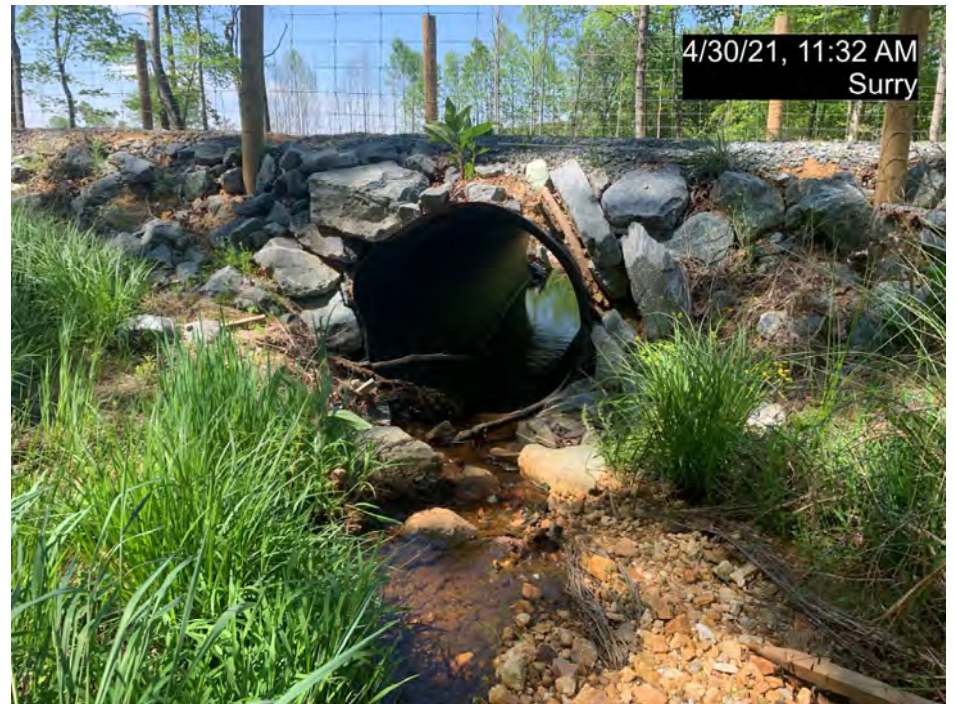
PS-3, R4, Culvert Crossing, Downstream (MY-02)
