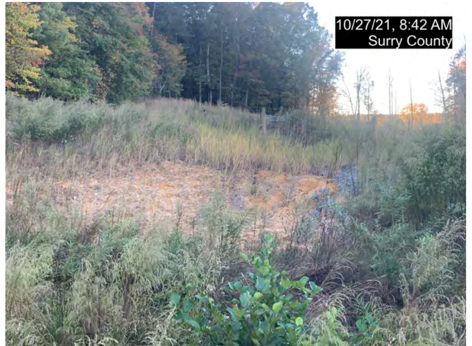
SPA4, R2 Right Floodplain, Minor Erosion (MY-02)
