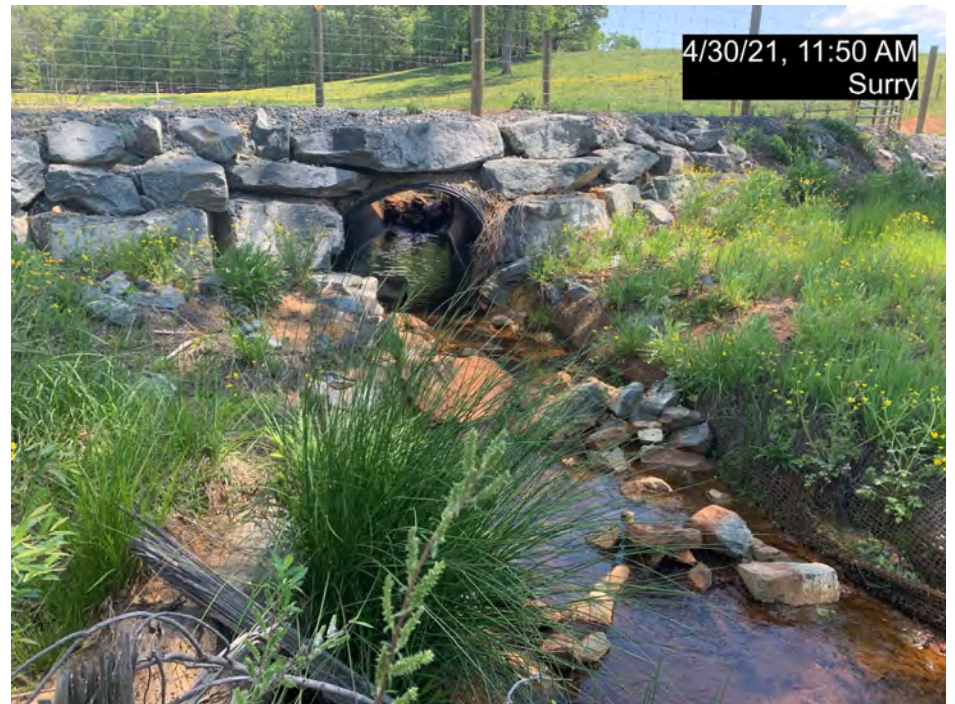
PS-6, R5, Culvert Crossing, Upstream (MY-02)
