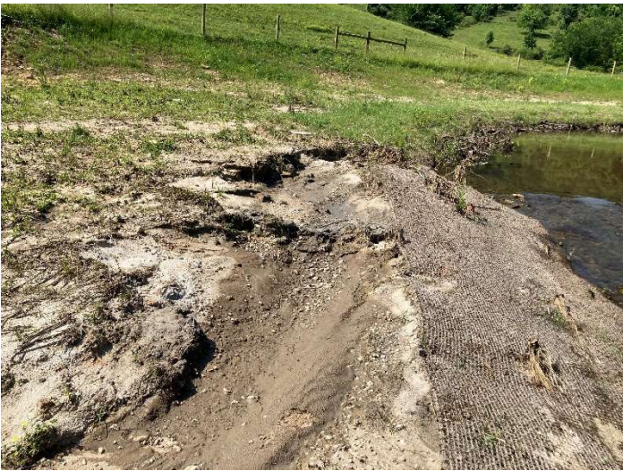
NL Hunting Reach 1, station 102+50 – Bank scour before repairs (6/1/2022)
