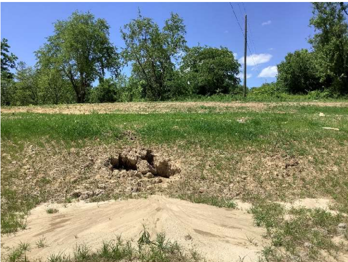
NL Hunting Reach 1, station 102+50 – Floodplain scour before repairs (5/24/2022)
