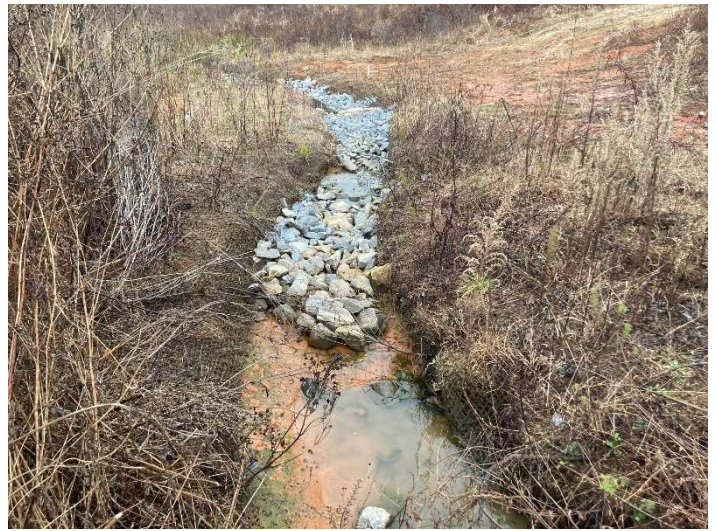
UT1 Reach 1, station 210+50 to 212+00 – Restabilized riffle after repairs (12/8/2022)
