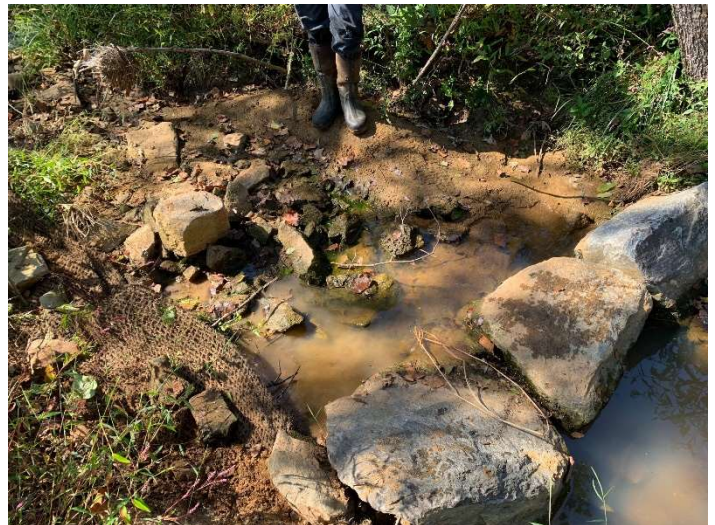
UT1 Reach 3, station 218+15 - Structure piping (10/5/22)
