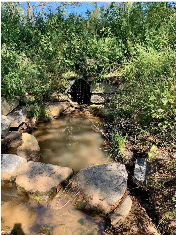
NCDWR Comment 1 (Erin Davis) – Ingle Hollow Road Culvert – Stream flow is piping around the sill and lowering the water surface elevation at the culvert's outlet (09/27/2022).
