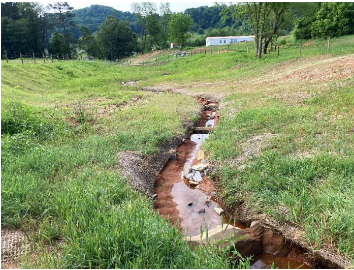
UT1 Reach 1, station 210+50 to 212+00 – Riffle scour before repairs (6/1/2022)
