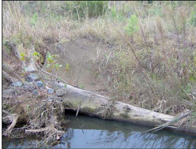
Piping at Log Vane on Wallace Branch, STA 29+50 10/24/08
