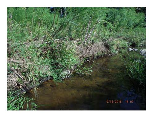
Headcut forming on bank in the middle mainstem. Downstream view.
