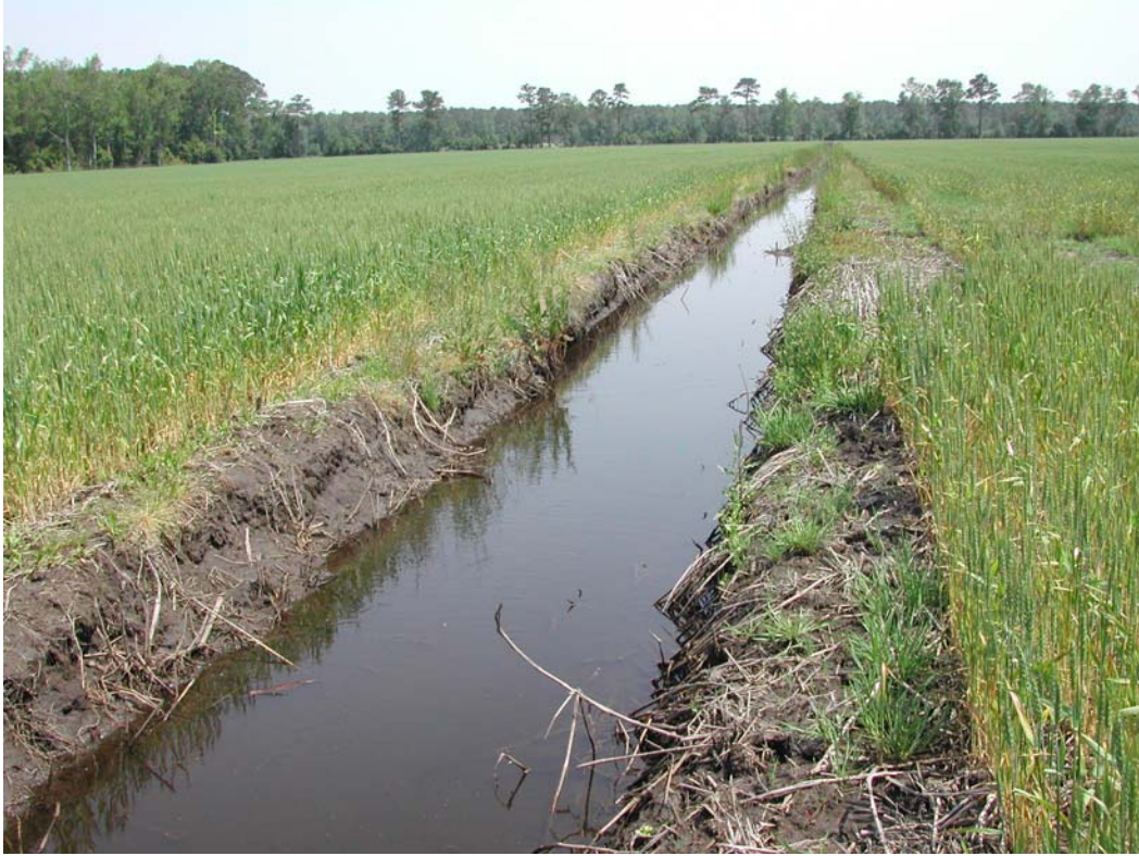
Photo 3. “Mason Ditch” with crops planted to edge pre-construction.
