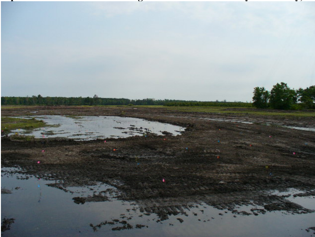
Photo 8. Successful wetland hydrology evident just after completion of construction. May, 2007
