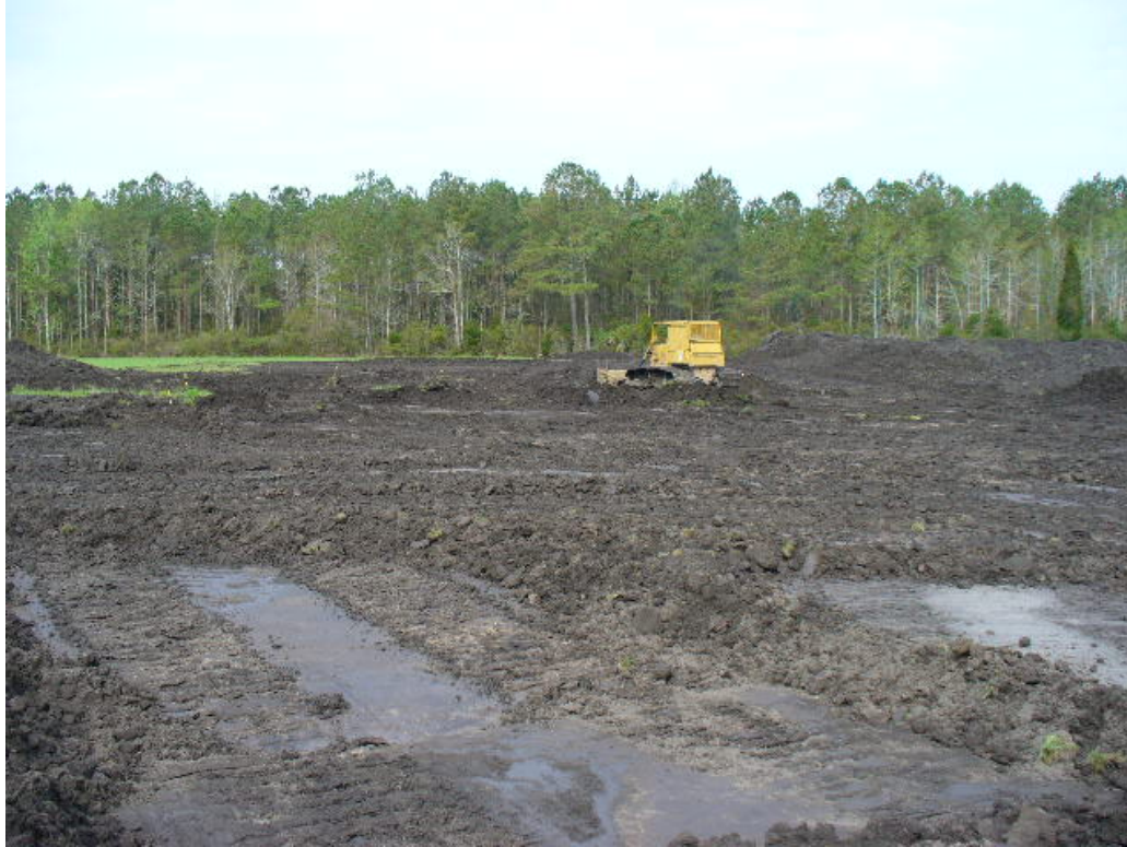
Photo 5. Wetland hydrology evident during construction. April, 2007
