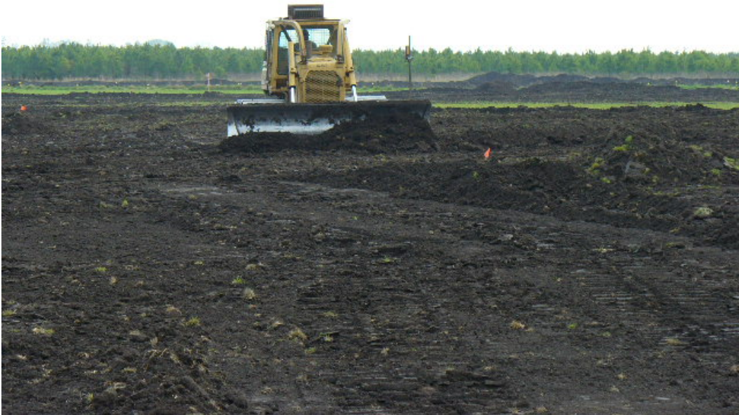
Photo 4. Deep organically rich soils encountered throughout the site during construction.
