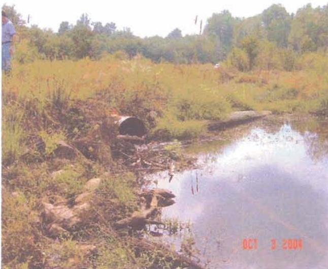
Upstream face of the 72 inch metal culvert – currently restricted to one half it's capacity.
