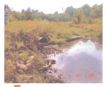
Upper ream face of the 72 inch metal culvert – currently restricted to one half it's capacity.
