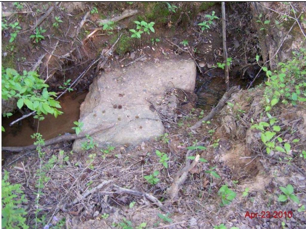
SPA8 UT5 Sta. 515+80 – Grade Control Degradation
