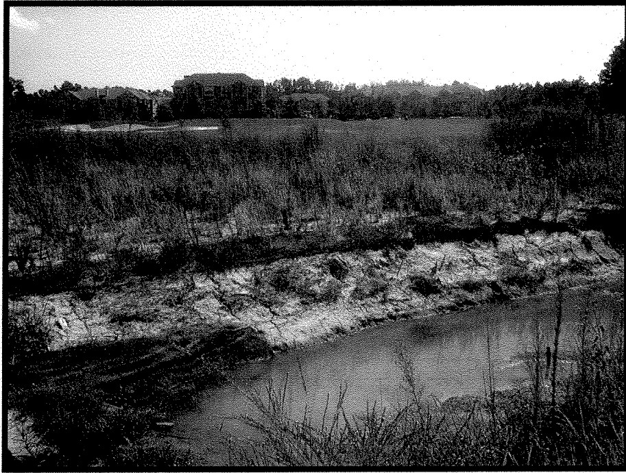
Vegetative Problem Area—Bare Bank
