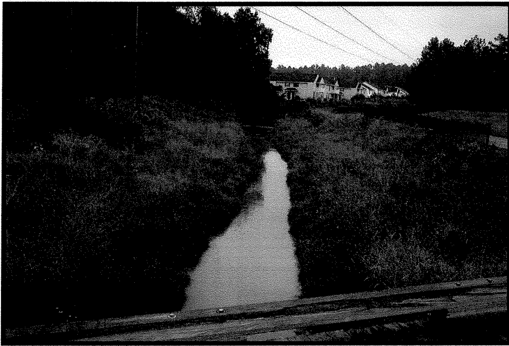
Lower 300 feet of restoration—As-built
