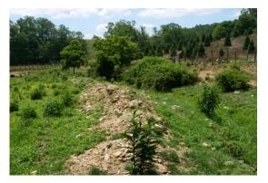
Sink Hole Creek Reach 1 berm formed by dredge spoils
