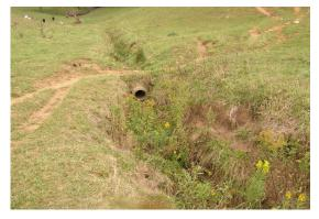
Pipe to be removed with incision and headcut on UT3
