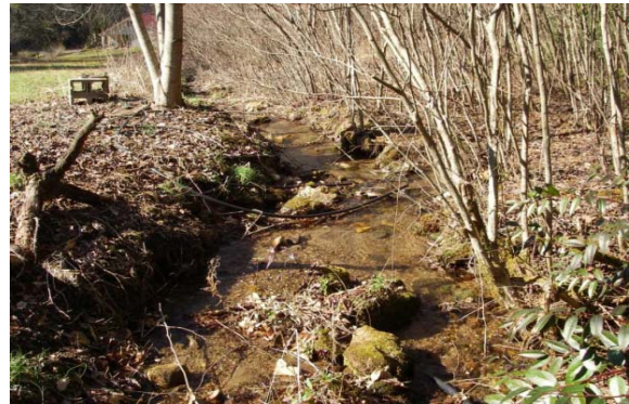
New alignment of UT3 would begin in the vicinity of location shown
