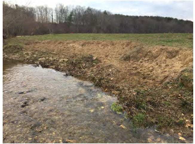
Moores Fork – Reach 2 with bank erosion from cattle access.
