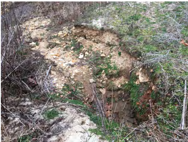
Moore's Fork – Reach 1 headcut at field drainage ditch.
