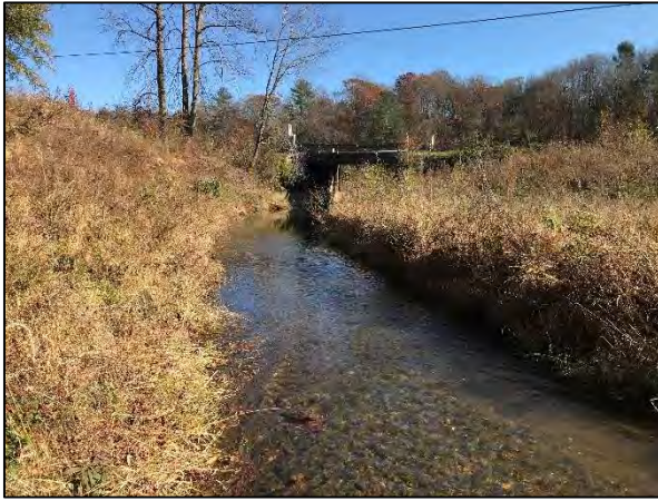
Photo Point 11B – Moores Fork Reach 2, Sta. 45+79 Facing Downstream (11/16/2021)
