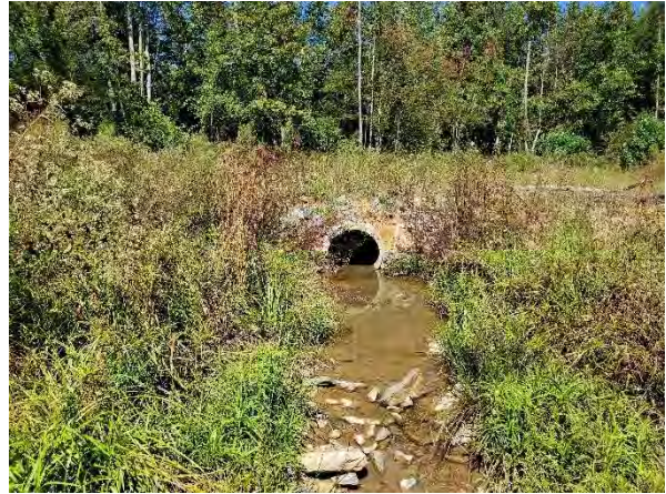
UT3 Culvert Opening (2021)
