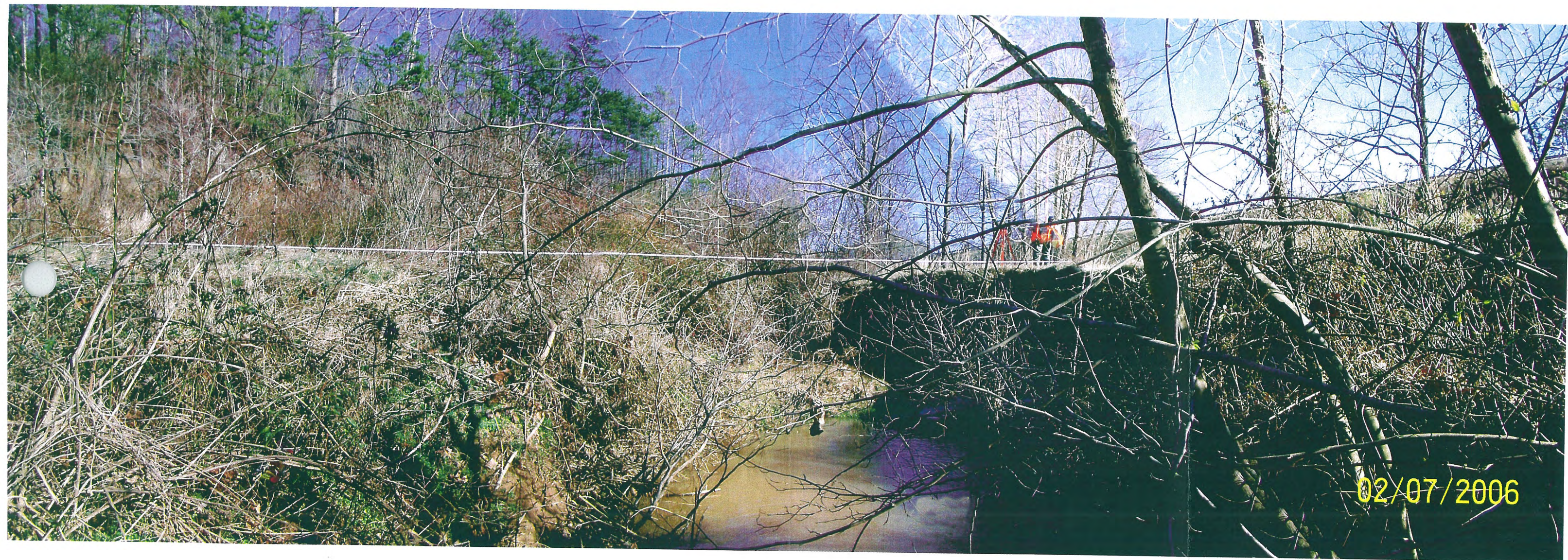
Thompsons Fork Mainstem Existing Conditions Pool Cross-Section Looking Down Stream near Confluence of Unnamed Tributary February 7, 2006
