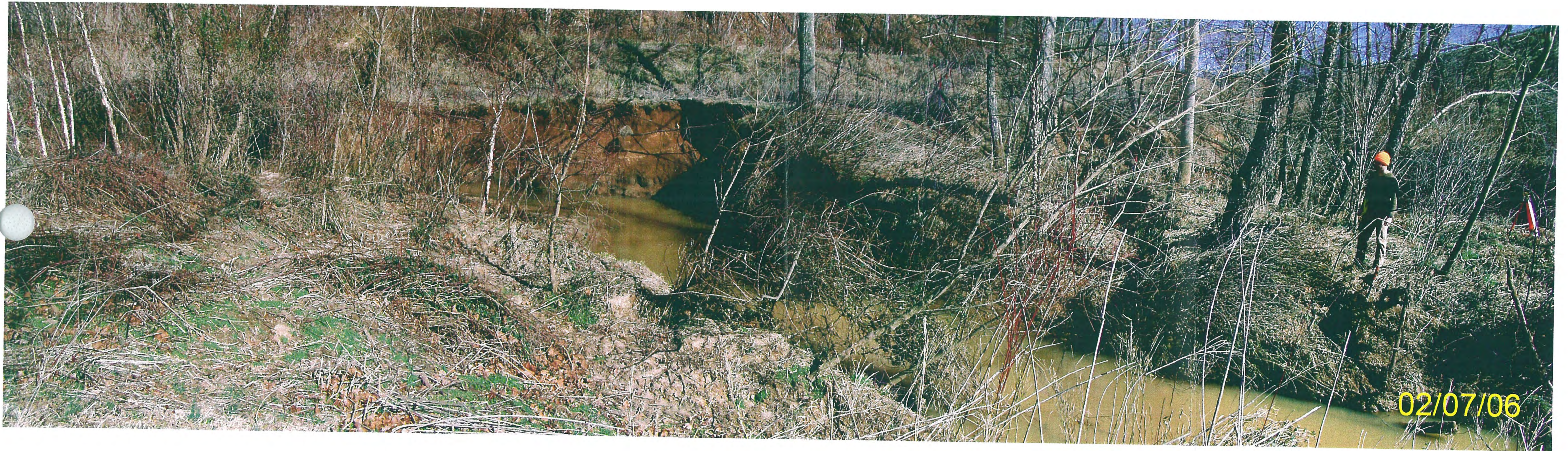
Down Stream Limits of Project Thompsons Fork Mainstem 15-ft Vertical to Undercut Streambank February 7, 2006
