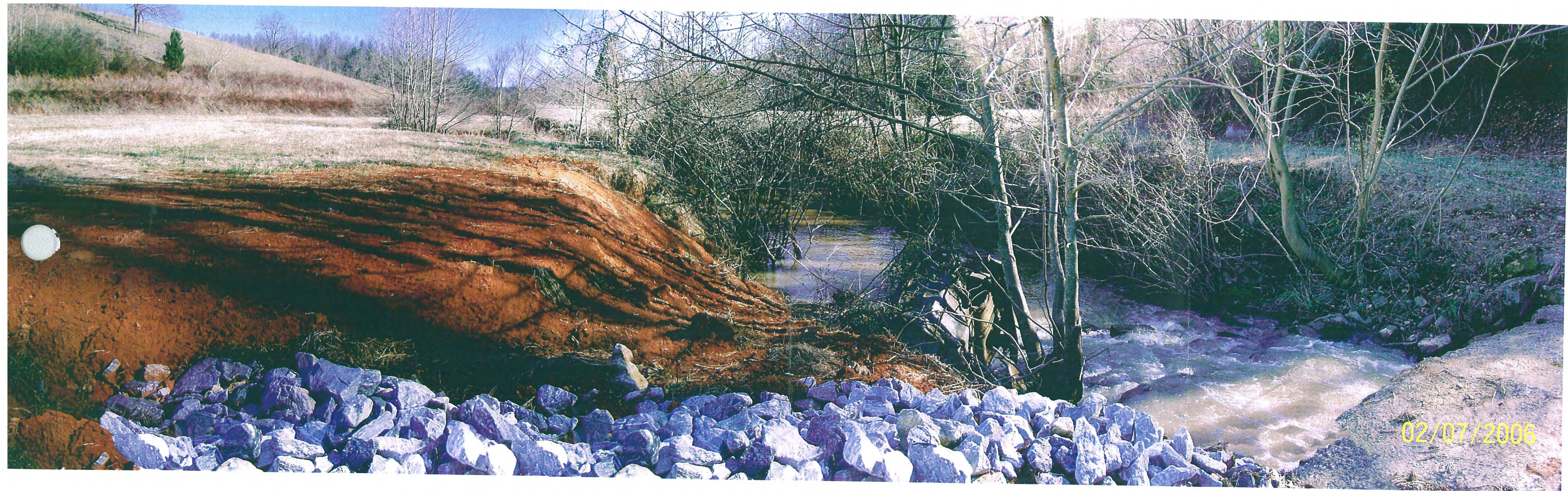
Existing Stream Crossing Thompsons Fork Mainstem Looking Down Stream February 7, 2006
