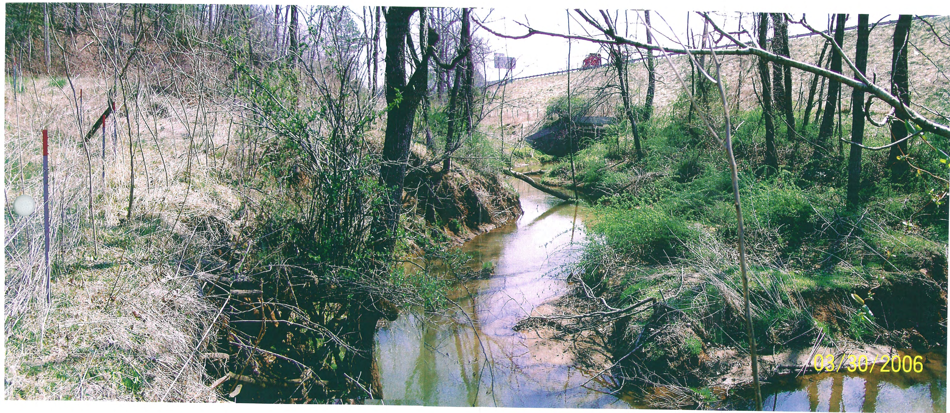
Thompsons Fork Mainstem End of Priority Level I Project Confined by South Creek Road & I-40 Inlet 3-Chamber Box Culvert Under I-40 March 30, 2006
