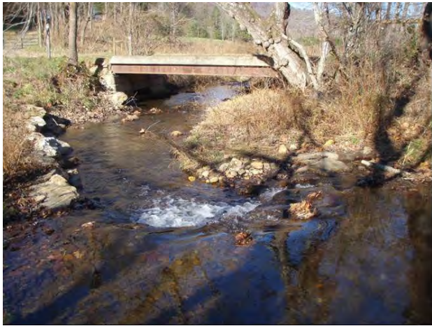
J-hook sta. 12+75, lower end of Bura/Roberson properties, 20 November 2012.
