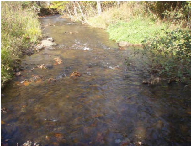
Cross vane, riffle construction, and bank shaping, sta. 6+75, 29 October 2013.
