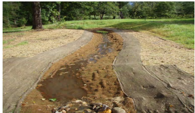
UT2 restored portion, east of Canterfield Lane, 5 September 2011.
