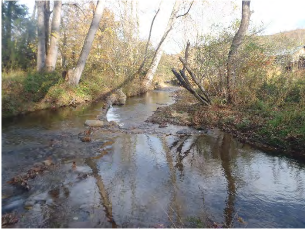
J-hook, sta. 2+50, facing downstream, 12 November 2014.
