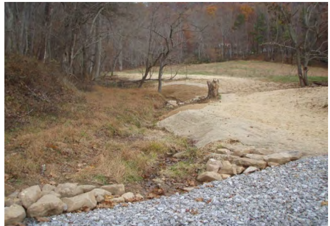
UT3 above ford, invasive removal, cattle exclusion, and bank shaping, facing upstream, 9 November 2011.
