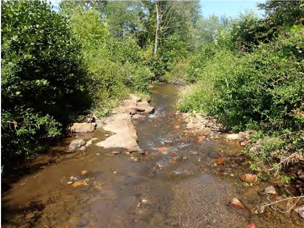
Bank sloping and J-hook, sta. 9+25 to 10+00, 15 September 2016.
