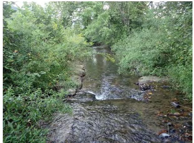
Cross vane, riffle construction, and bank shaping, sta 6+75 15 September 2016.
