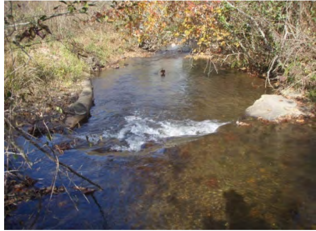
Log vane, root wads, and bank shaping, sta. 4+50, facing downstream 29 October 2013.
