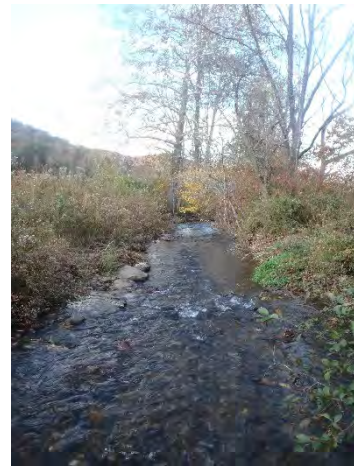
Cross vane, riffle construction, and bank shaping, sta. 6+75, 12 November 2014.
