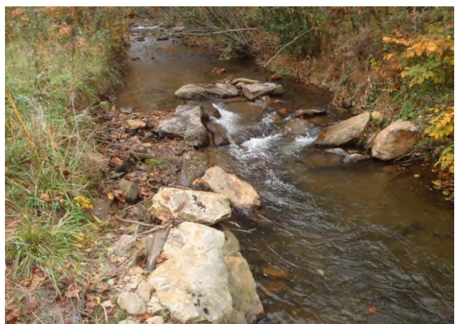
Rock vane, sta 1+50 facing upstream, 28 October 2014
