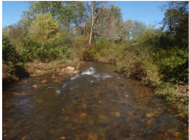
Bank sloping and J-hook, sta. 9+25 to 10+00, 23 November 2015.
