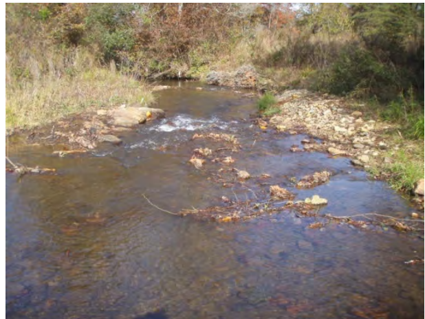
Bank sloping and J-hook, sta. 9+25 to 10+00, 29 October 2013.
