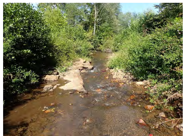
Aggradation and bar formation below J-hook, sta. 9+25 to 9+50, following 5 May 2013 flood event, facing downstream, 12 September 2016.
