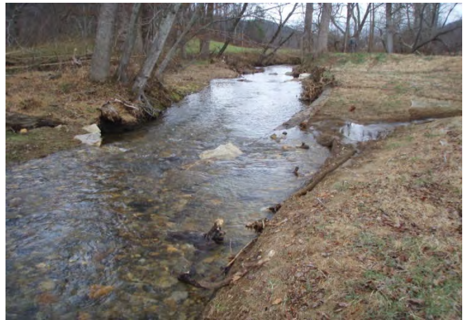
Log vane sta. 1+00 to 1+50, facing downstream
