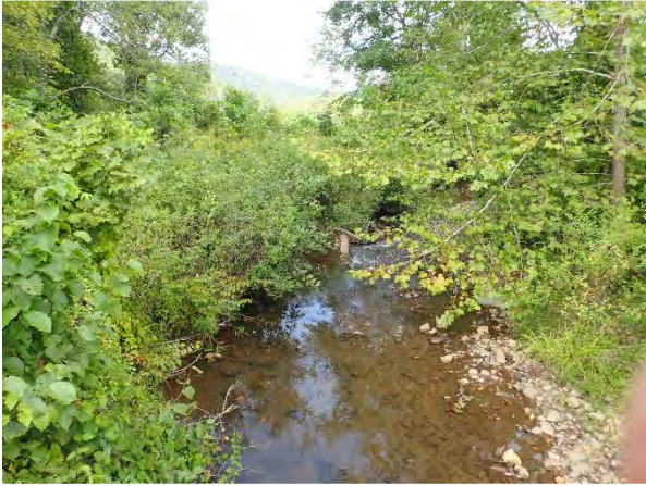
Bank shaping, log vane, and riffle construction, sta. 0+25, 15 September 2016
