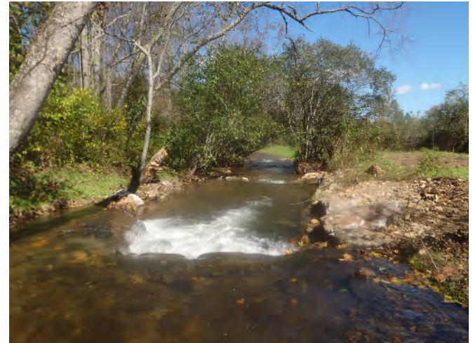
Crossvane after summer 2015 repairs, facing downstream, sta. 0+50, 14 October 2015
