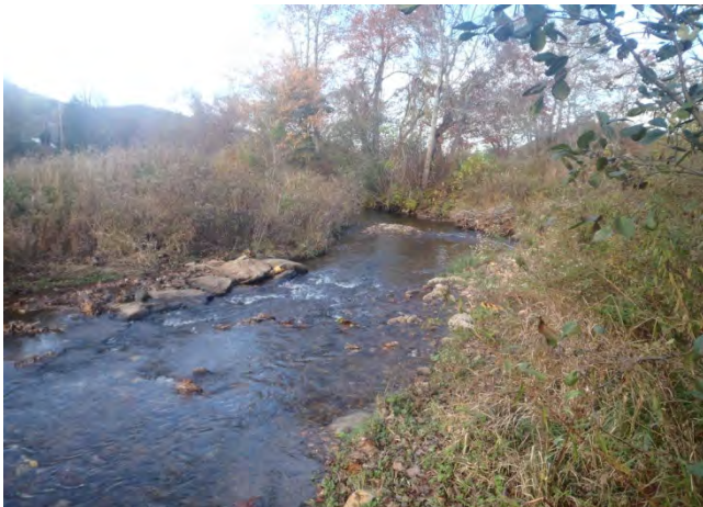
Bank sloping and J-hook, sta. 9+25 to 10+00, 12 November 2014.
