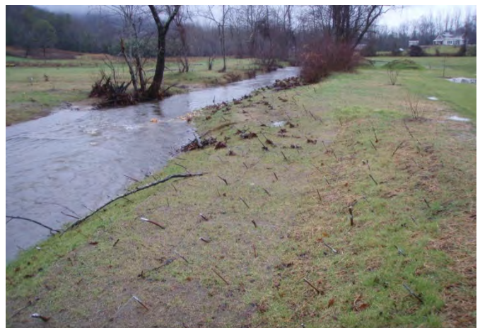
Log vane, root wads, and bank shaping, sta. 2+25 to 3+50, facing downstream, 7 December 2011.
