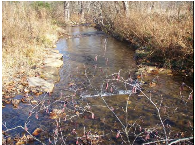
Cross vane, riffle construction, and bank shaping, sta. 6+75, 20 November 2012.
