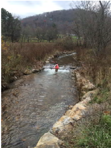
Repaired J-hook, sta. 12+75, facing upstream, 15 October 2015
