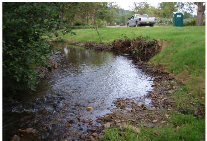
Bank shaping, root wads, and toe-wood, sta. 11+50 to 12+00, facing downstream, 22 September 2011.
