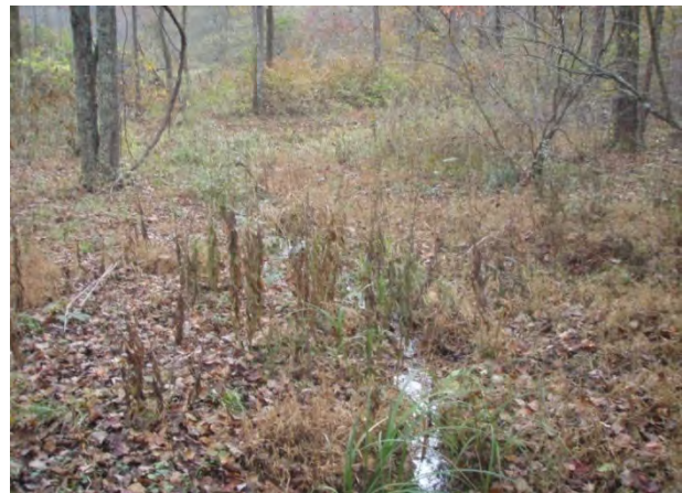
UT1 Priority I construction, above vernal pond, 29 October 2013.
