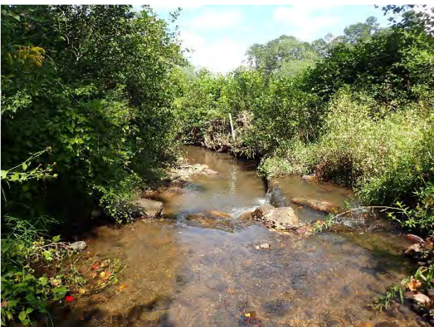
Log vane, root wad, and bank shaping, sta. 7+25 to 8+00, 15 September 2016.
