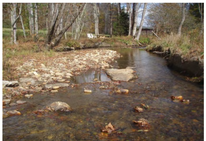
J-hook, sta. 2+50, facing downstream, 29 October 2013.
