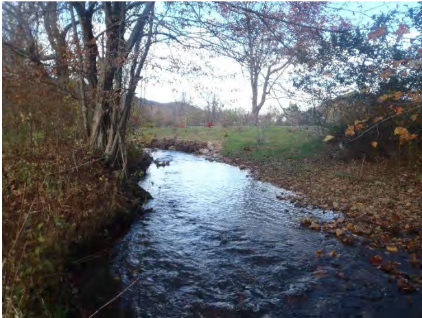
Bank shaping, root wads, and toe-wood, sta. 11+50 to 12+00, facing downstream, 12 November 2014.
