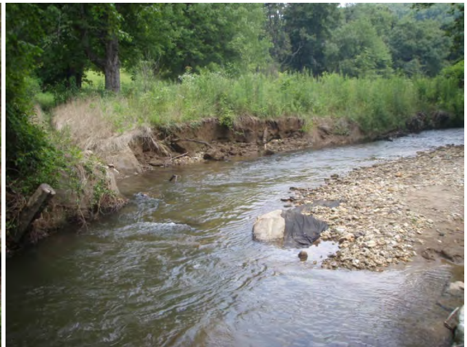
Right bank scour and erosion during 5 May 2013 flood event, facing upstream, sta. 12+50, 18 July 2013.
