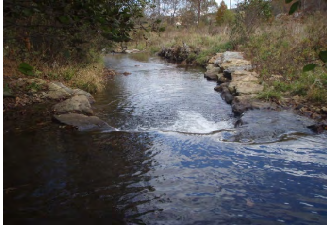
J-hook, sta. 5+00, facing downstream, 29 October 2013.
