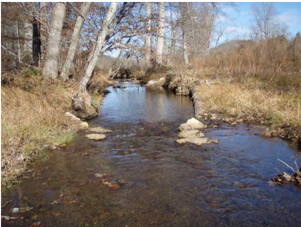
Log vane sta. 1+00 to 1+50, facing downstream, 20 November 2012.
