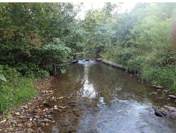
Log vane, root wads, and bank shaping, sta. 4+50, facing upstream 15 September 2016.
