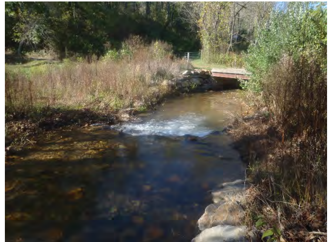
Repaired J-hook, sta. 12+75, facing downstream, 14 October 2015
