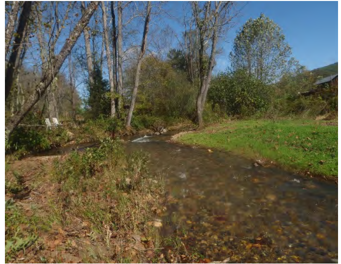
Meander below J-hook sta 2+50 after summer 2015 repairs facing downstream 14 October 2015 No longer considered a problem during MY4 (2015) field surveys.
