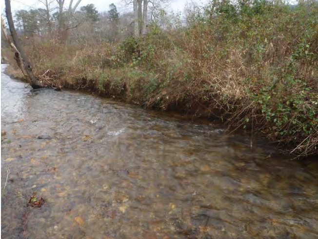
Right bank erosion due to high flow events, sta. 5+05 to 6+10 facing downstream, 17 November 2015.
