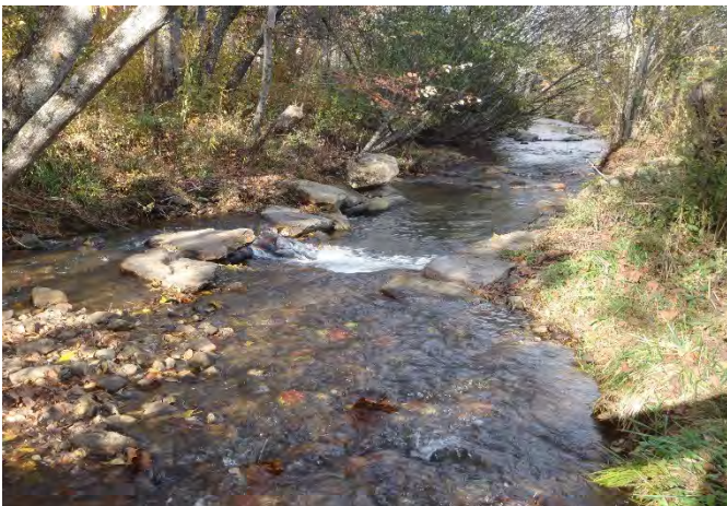
Cross vane, sta. 0+50, facing downstream, 12 November 2014.
