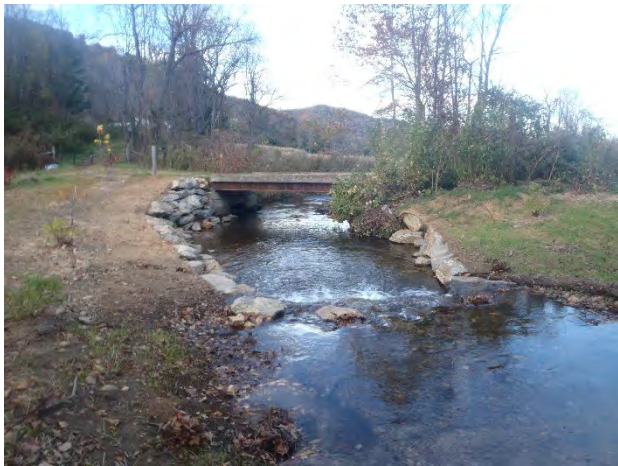
J-hook sta. 12+75, lower end of Bura/Roberson properties, 12 November 2014.
