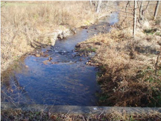
Bank shaping, log vane, and riffle construction, sta. 0+25, 20 November 2012.
