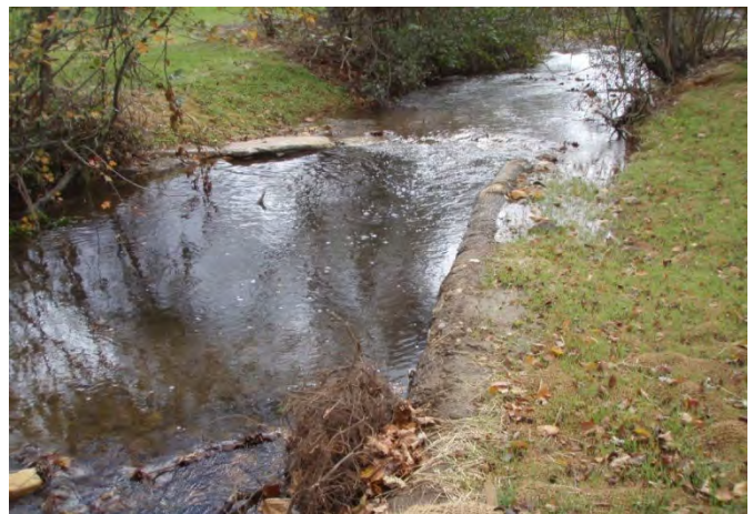
Log vane, root wads, and bank shaping, sta. 4+50, facing upstream, 19 October 2011.
