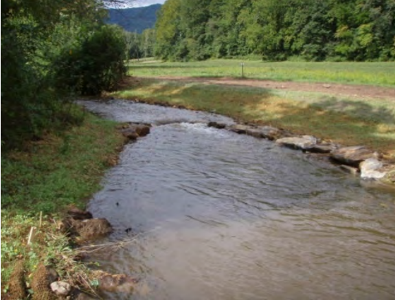
J-hook vane after construction, sta. 9+25, facing upstream, 5 September 2011.
