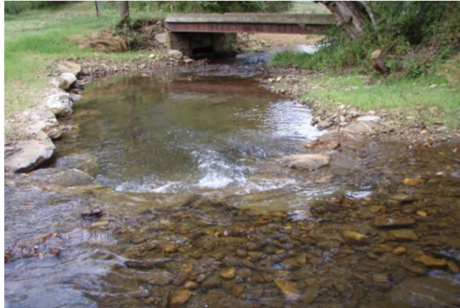
J-hook sta. 12+75, lower end of Bura/Roberson properties, 22 September 2011.
