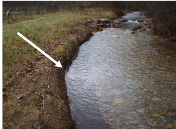
Right channel bank instability after flood damage, sta. 1+75 to 2+25, facing upstream, 5 December 2011.
