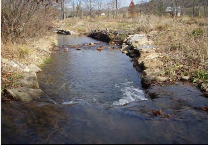
J-hook, sta. 5+00, facing downstream, 20 November 2012.
