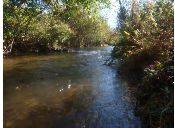
Log vane, root wads, and bank shaping, sta. 4+50, facing upstream 14 October 2015.
