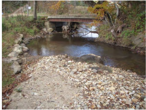
J-hook sta. 12+75, lower end of Bura/Roberson properties, 29 October 2013.
