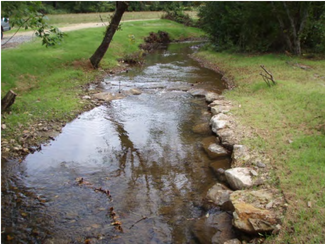
J-hook, sta. 12+75, after construction, facing upstream, 22 Sept 2011.
