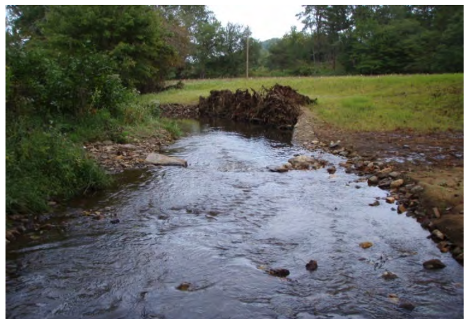
Log vane, root wad, and bank shaping, sta. 7+25 to 8+00, 22 September 2011.
