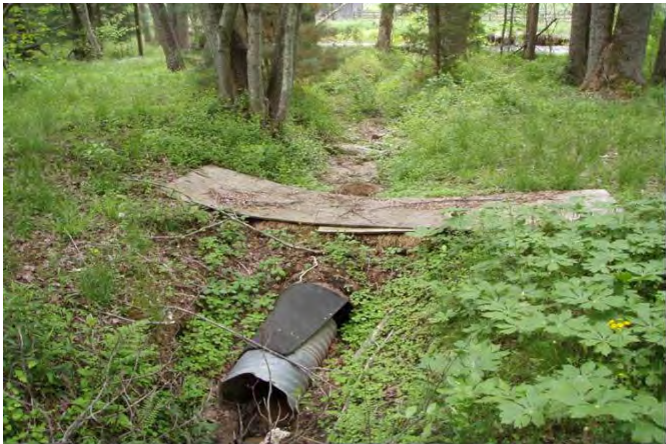
UT1 facing downstream, pre-construction 28 July 2009.
