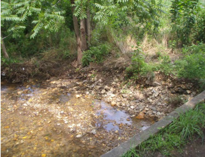
Right bank scour during 5 May 2013 flood event, sta. 0+00 to 0+20, facing downstream, 18 July 2013.
