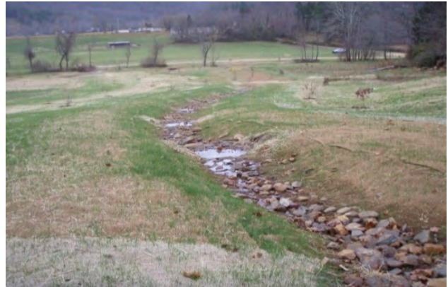
UT3 below ford, Priority I channel restoration, facing downstream, sta. 0+00, 15 November 2011.
