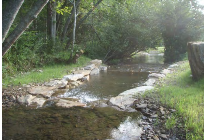
Cross vane, sta. 0+50, facing downstream, 14 August 2011.
