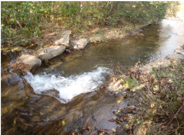
J-hook, sta. 5+00, facing downstream, 12 November 2014.
