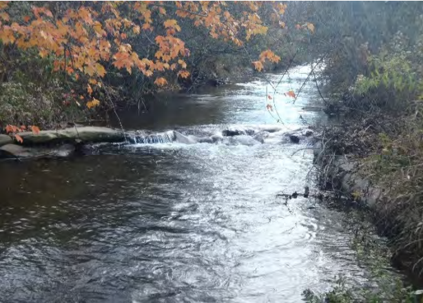
Log vane, root wads, and bank shaping, sta. 4+50, facing upstream 12 November 2014.
