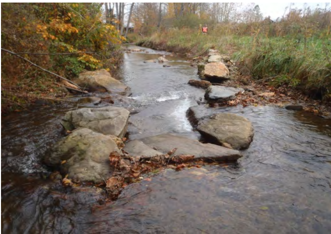
Rock vane, sta 1+50 facing downstream, 28 October 2014
