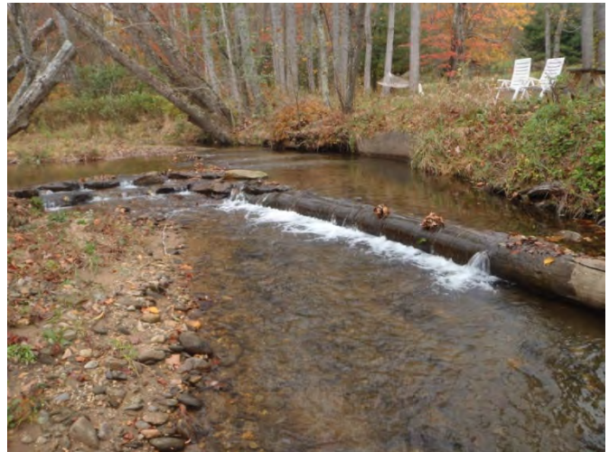
Aggradation below J-hook, sta 4+00 to 4+50, facing upstream, 28 October 2014
