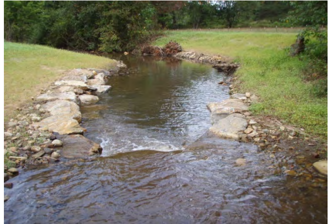
Bank sloping and J-hook, sta. 9+25 to 10+00, 22 September 2011.
