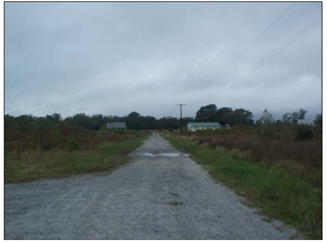
Photo Point 4 – 10/19/11 - MY 04 – Road Crossing Type A – Station 17+75 – Facing west toward Macedonia Road.
