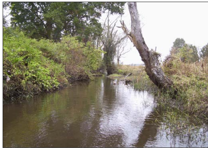
Cross-section 1, looking downstream
