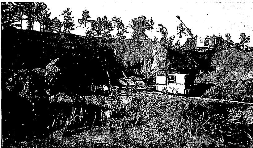
Fig. 5. Removing Overburden, Norlina Mining Company, Wood, N. C.
