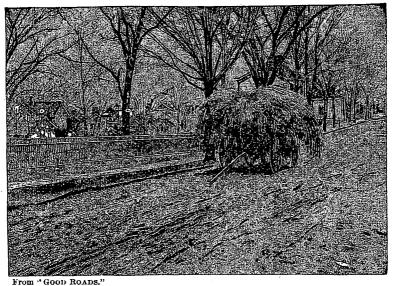
Fig. 6.—A LOAD OF HAY WHICH TWO LARGE HORSES WERE UNABLE TO PULL ON A MUDDY AMERICAN DIRT ROAD.
