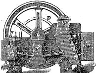
Fig. 39.-FARREL MARSDEN CRUSHER, SECTIONAL VIEW.
