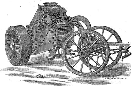
Fig. 40.-CHAMPION ROCK CRUSHER, PORTABLE VIEW.
