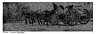
Fig. 2.—HEAVY LOAD OF STONE BEING HAULED ON A MACADAM ROAD. IT SHOULD BE OBSERVED THAT THE WHEELS DO NOT SINK INTO THE SURFACE, AND THAT CON-SEQUENTLY THE LOAD WHICH CAN BE HAULED IS GREATLY INCREASED.
