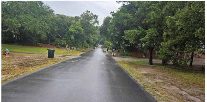
After: These observations confirm that the project successfully reduces flooding duration and volume, protecting the roadway and surrounding areas while improving stormwater management.
