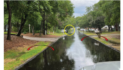
During 1.11 inches of rain, the swales working to get water off the road
