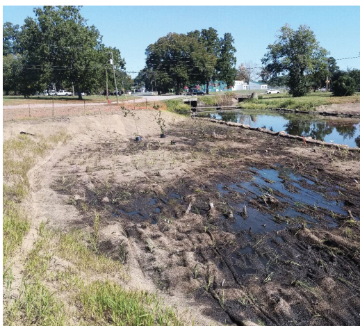
Jack's Creek Floodplain during construction
