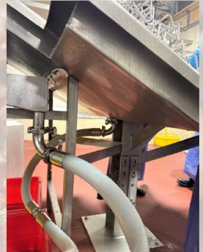
brine recovery hoses
