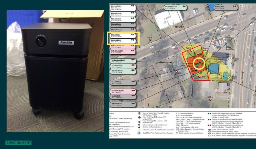
1. As an interim measure, we installed Air Purifying Units (APUs) to filter IA concentrations to acceptable non-residential worker concentrations / risk
