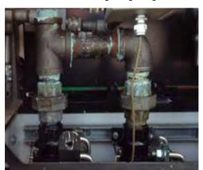
Figure 1: Improperly installed product pipe manifold above the shear valves
